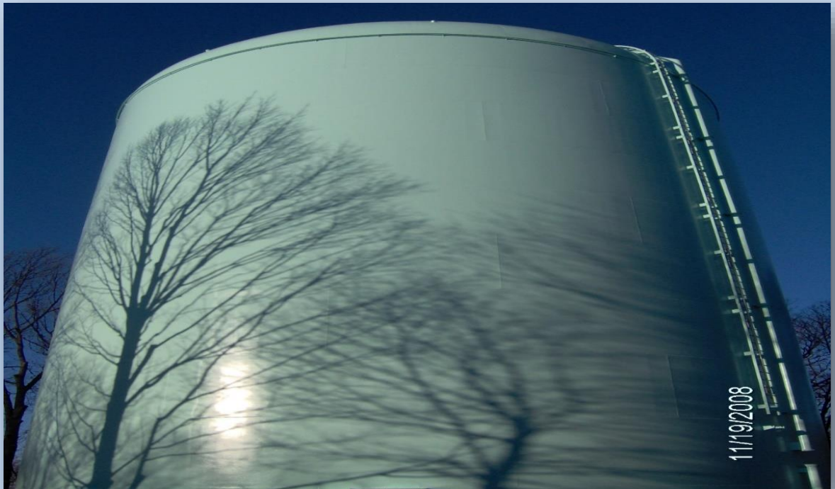
Dunster Road 1.5 Million Gallon Water Storage Tank
