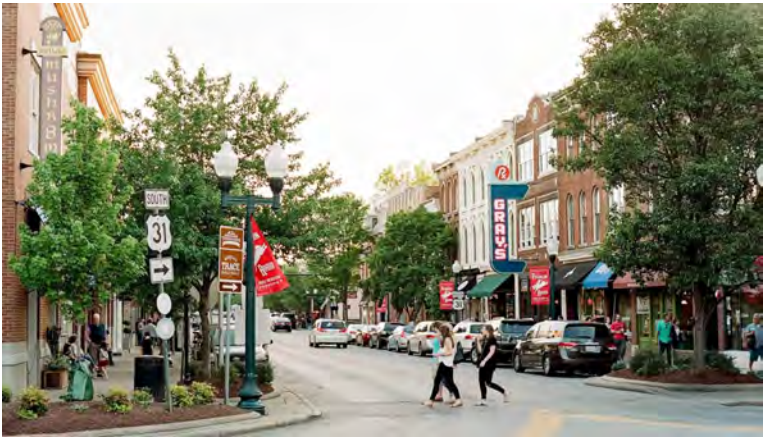
3-story MXU multifamily
