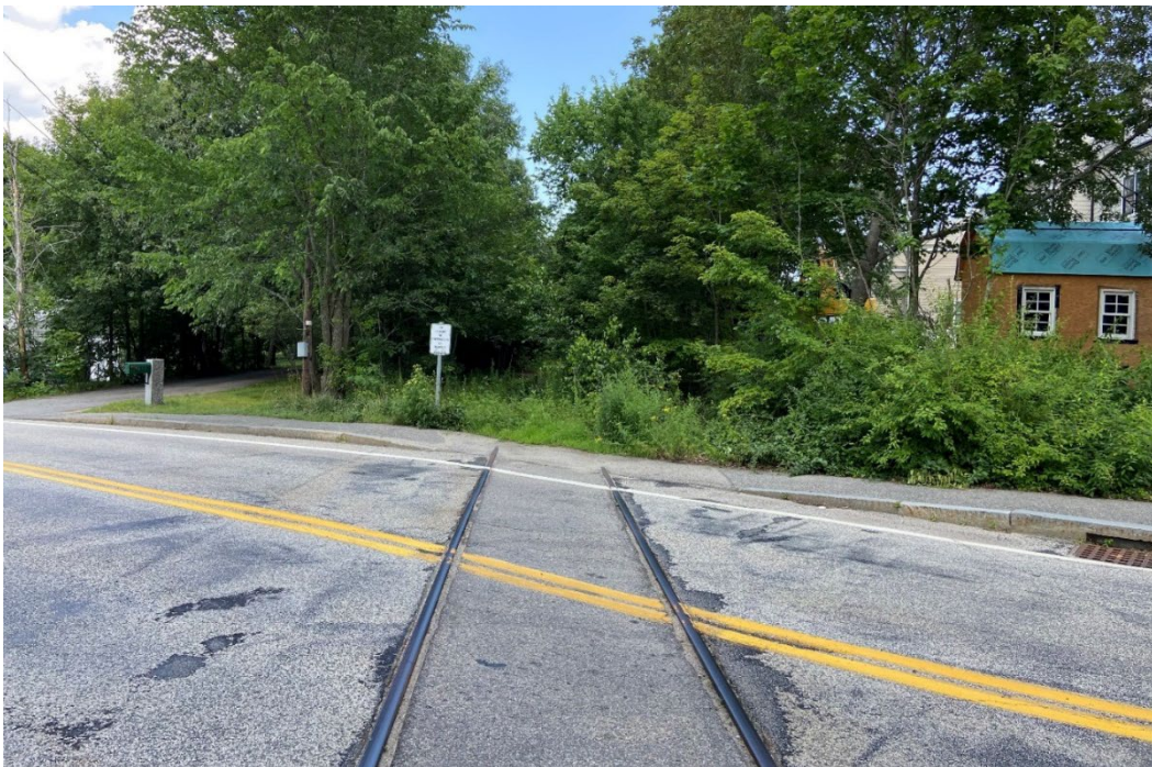
Photo 1: MBTA ROW crossing of Webster Street
