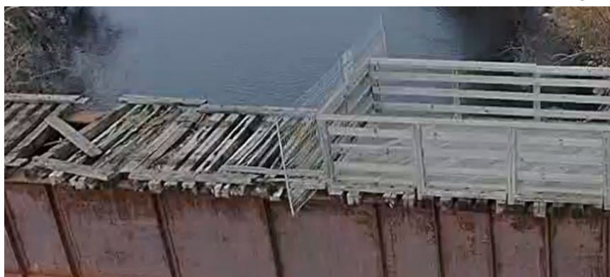
Photo 14: Existing Topside of Bridge
