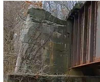
Photo 15: Existing South Bridge Seat
