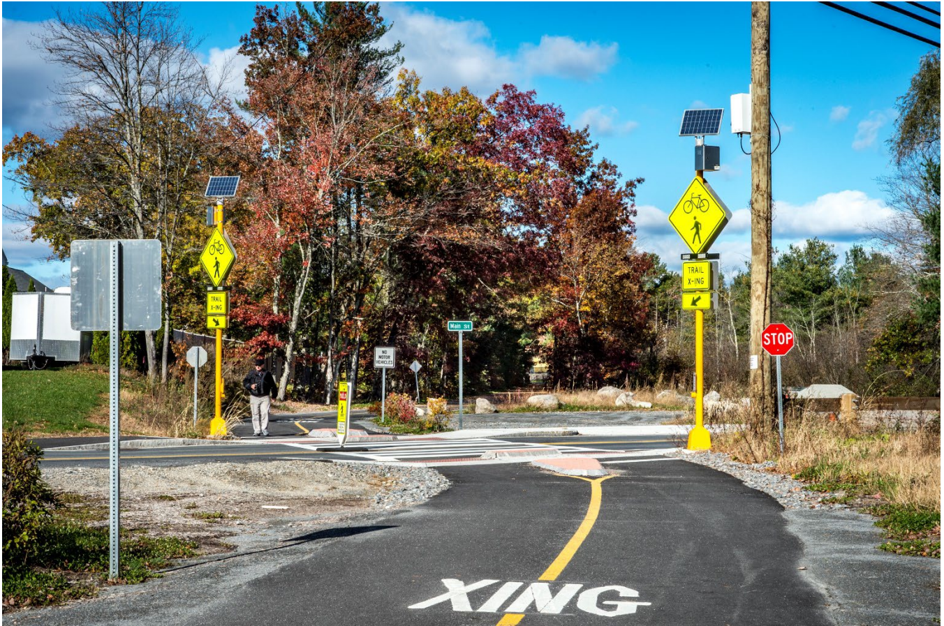
Photo 16 Bruce Freeman Rail Trail shared-use path crossing in Acton, with RRFB, signage, detectable warning plates and high visibility crosswalk.
