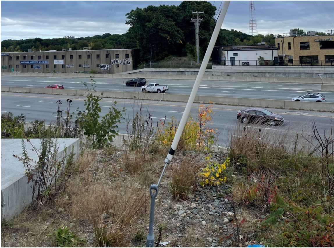
Photo 7: MBTA Right-of-Way at I-95 / Route 128
