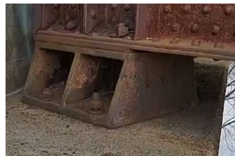
Photo 13: Condition of Bearings
