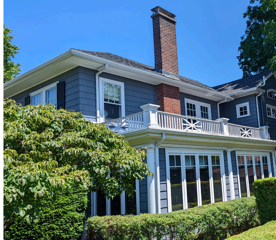
EXISTING RAILING STYLE
