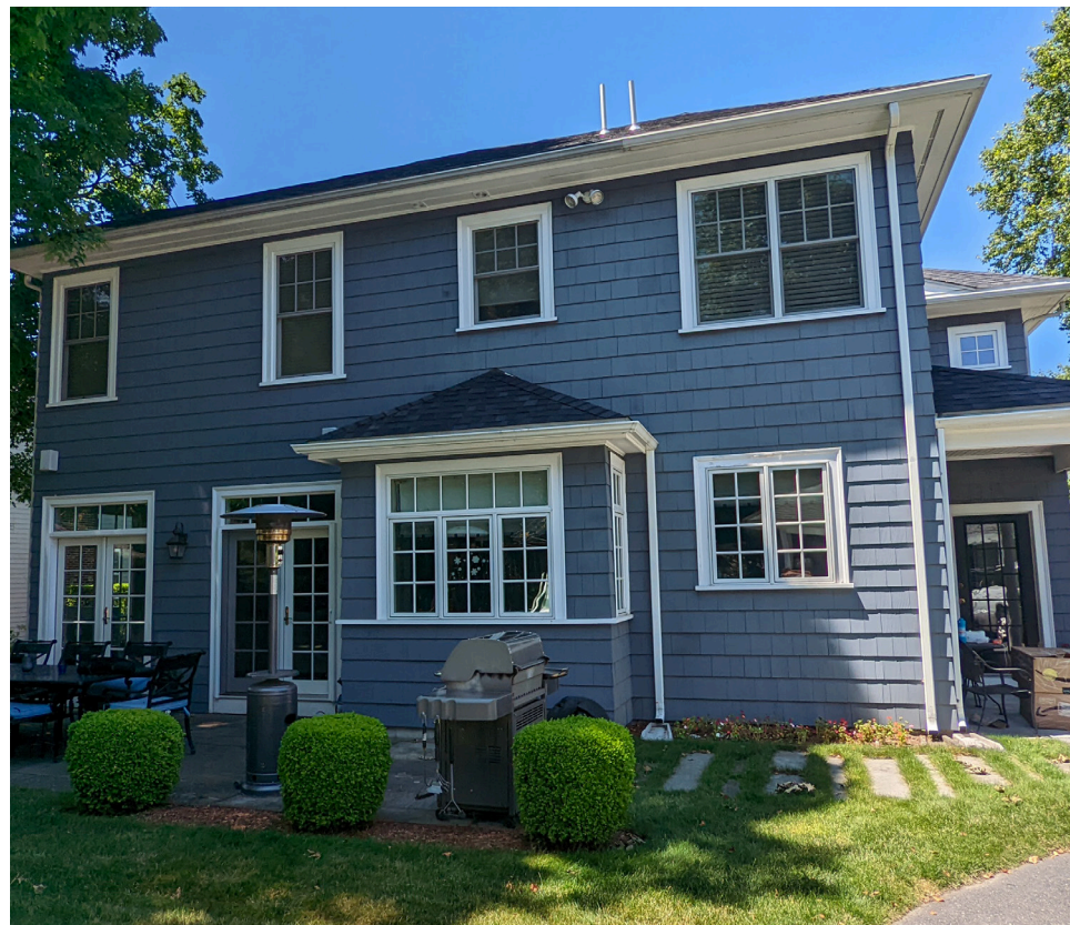
EXISTING REAR FACADE AND PATIO
