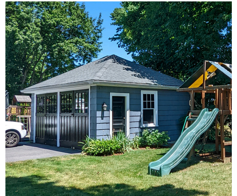
EXISTING GARAGE TO BE DEMOLISHED
