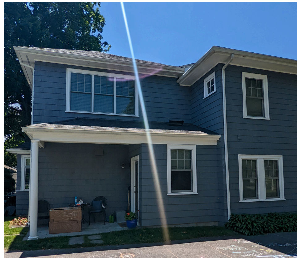
EXISTING MUDROOM ENTRY AND OFFICE ABOVE
