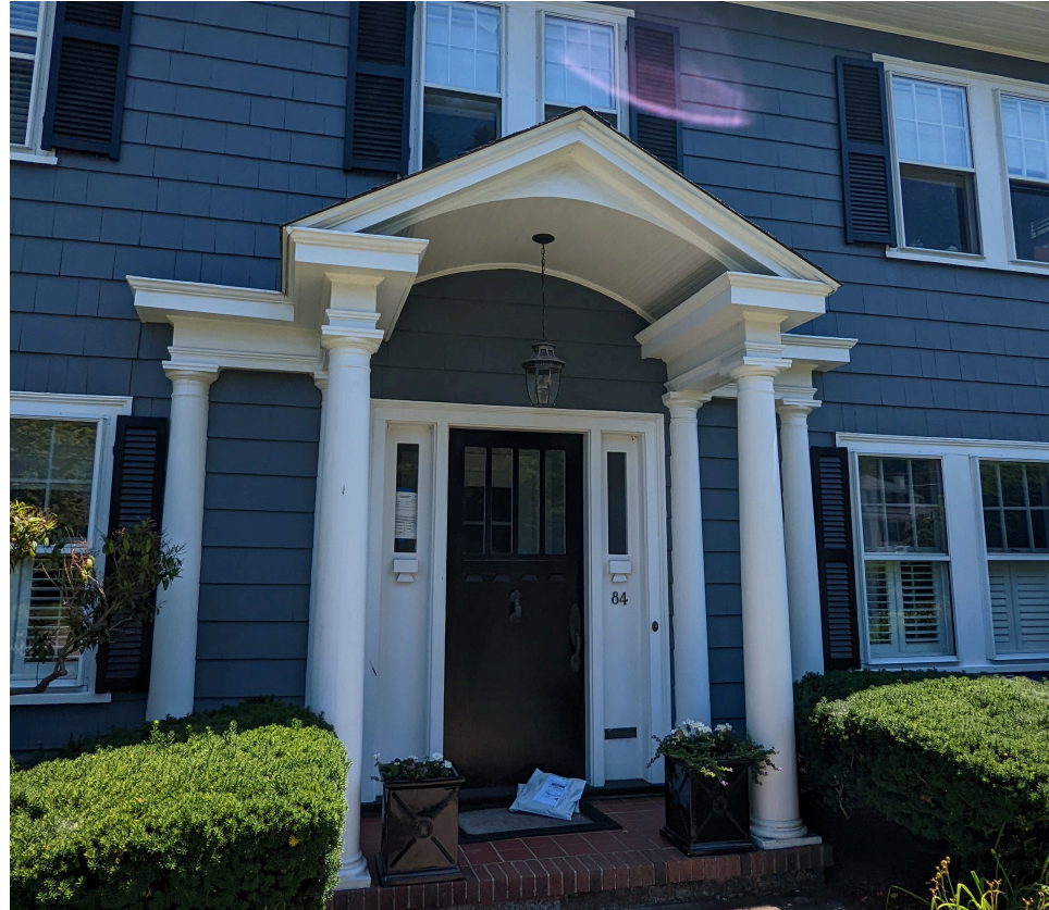
EXISTING FRONT ENTRY PORTICO
