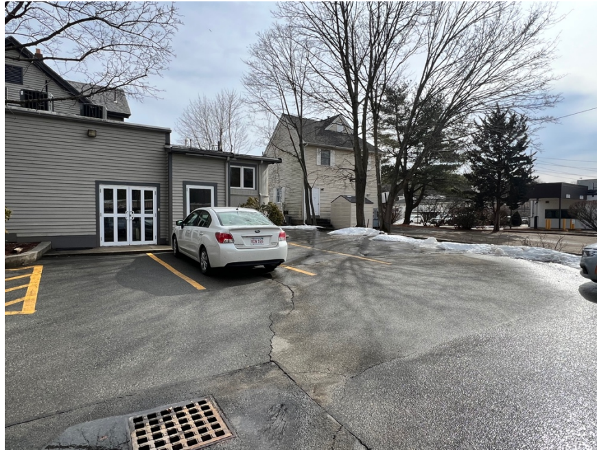
Back Parking Building Side
