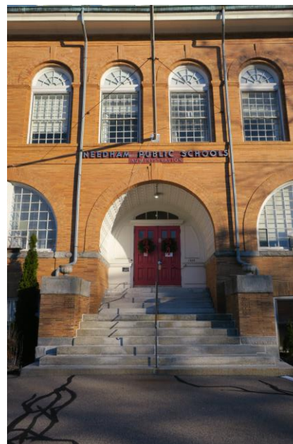
windows in these brick niches create useable office space
