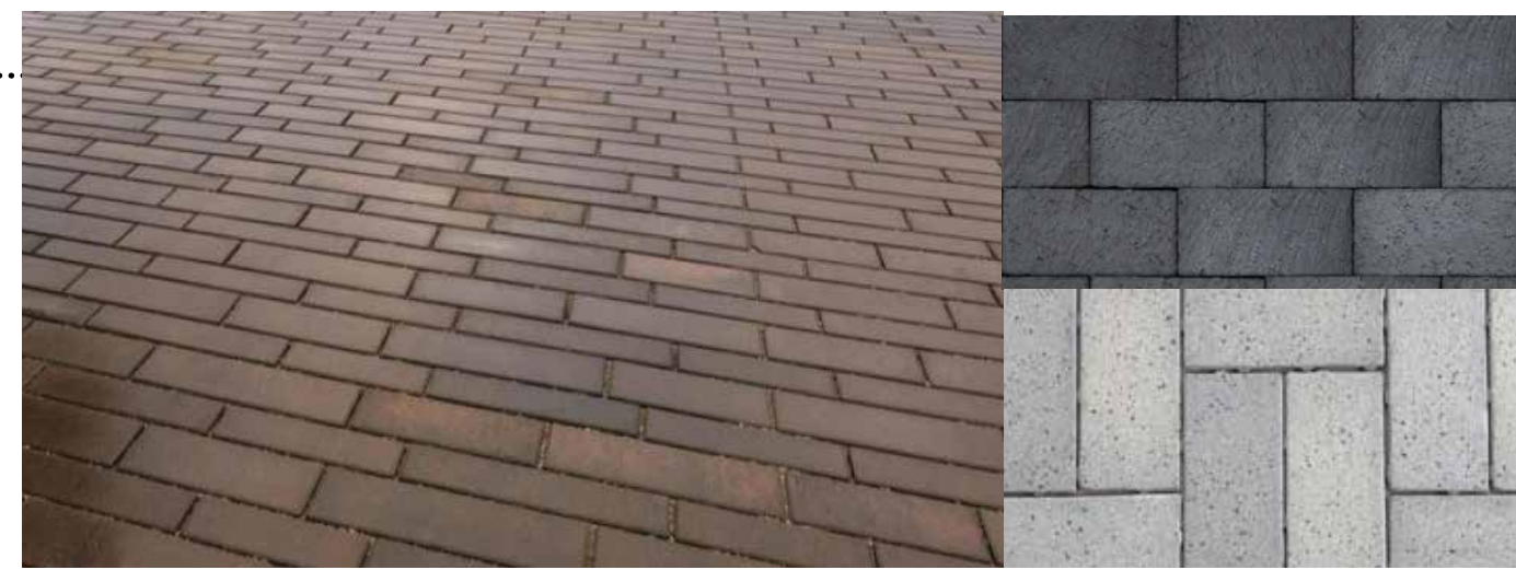
Precast Permeable Concrete Pavers - accent walk from HC parking with different colors.
