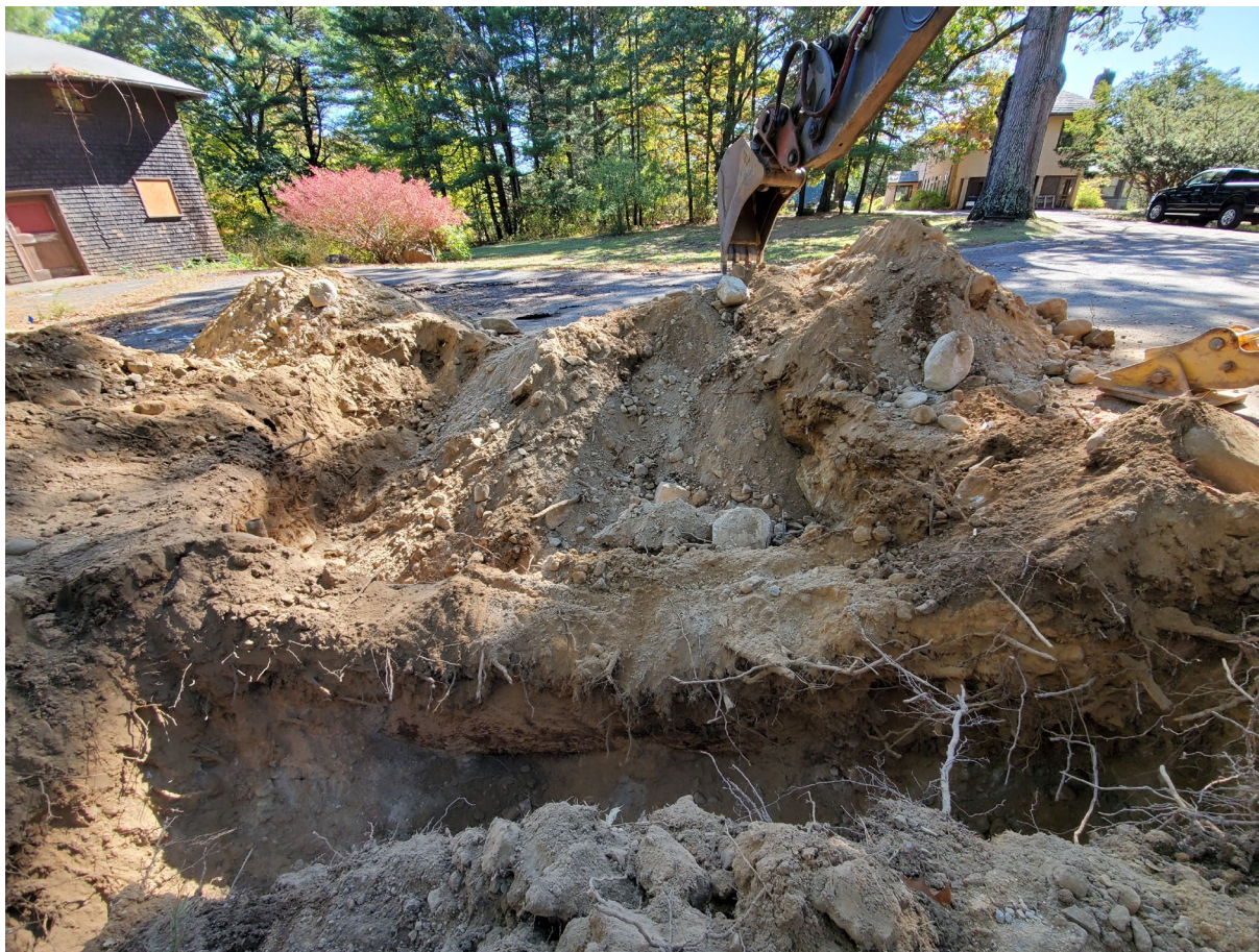
Photo 3: Facing east at the barn and underground storage tank
