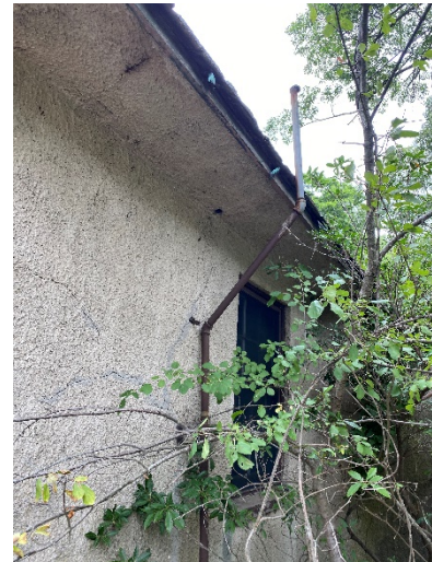
Fuel Tank Vent
