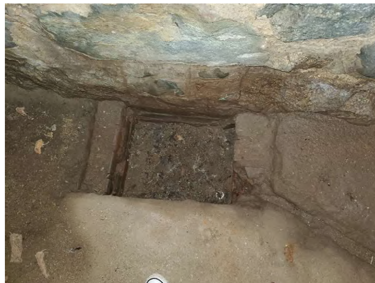
Photo #10: A drain located in the basement
