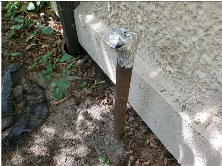
Photo #3: A vent pipe located in the front of the manor house
