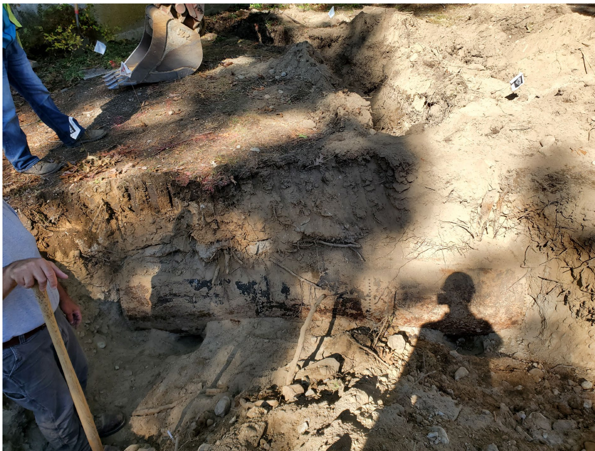
Photo 2: Facing west at the garage and underground storage tank
