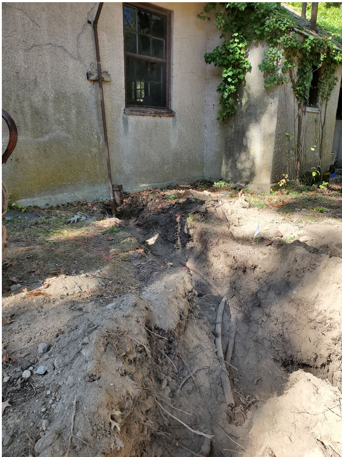
Photo 1: Facing west at the garage and (2) underground steel pipes
