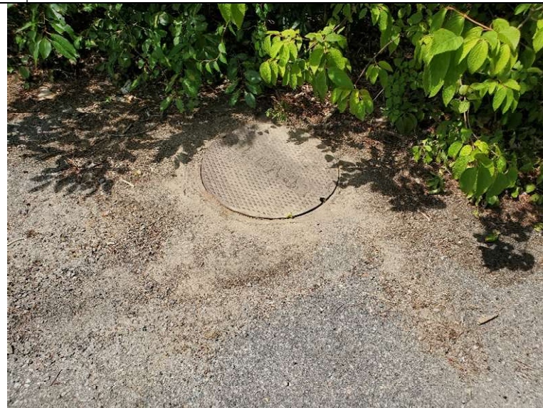
Photo #4: A sewer manhole cover located in front of the manor house
