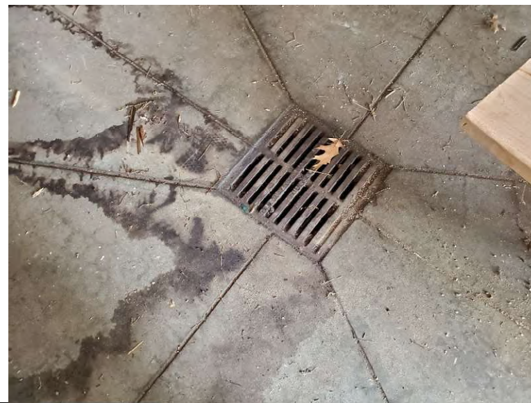
Photo #12: Floor drain in the garage
