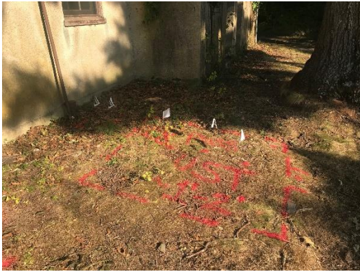
Picture 1: Closer look of “possible” tank location. The observed depth was between 1’ – 2’ below the surface.
