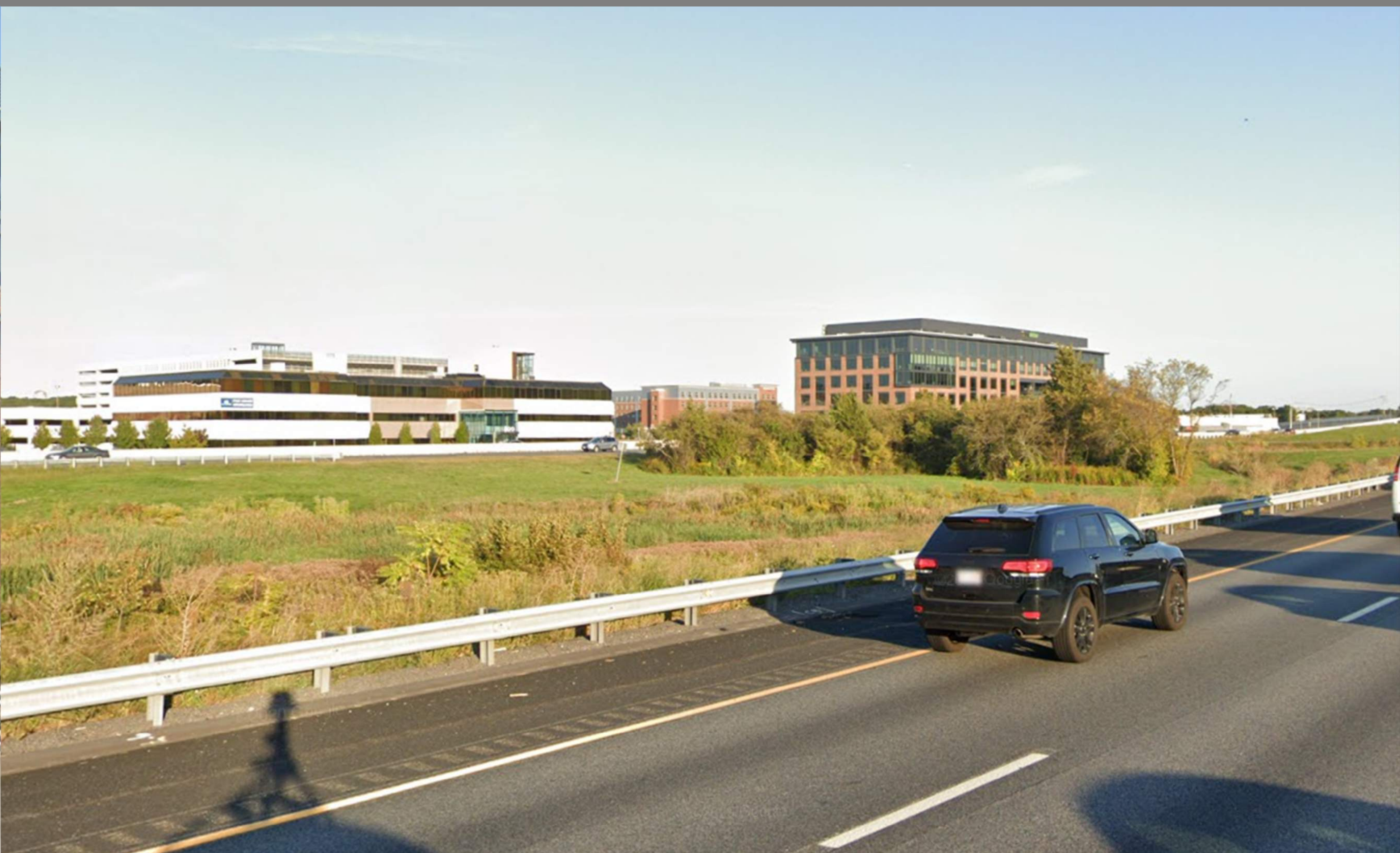
SITE VIEW - 128 FROM NORTH TRAVELING SOUTH
