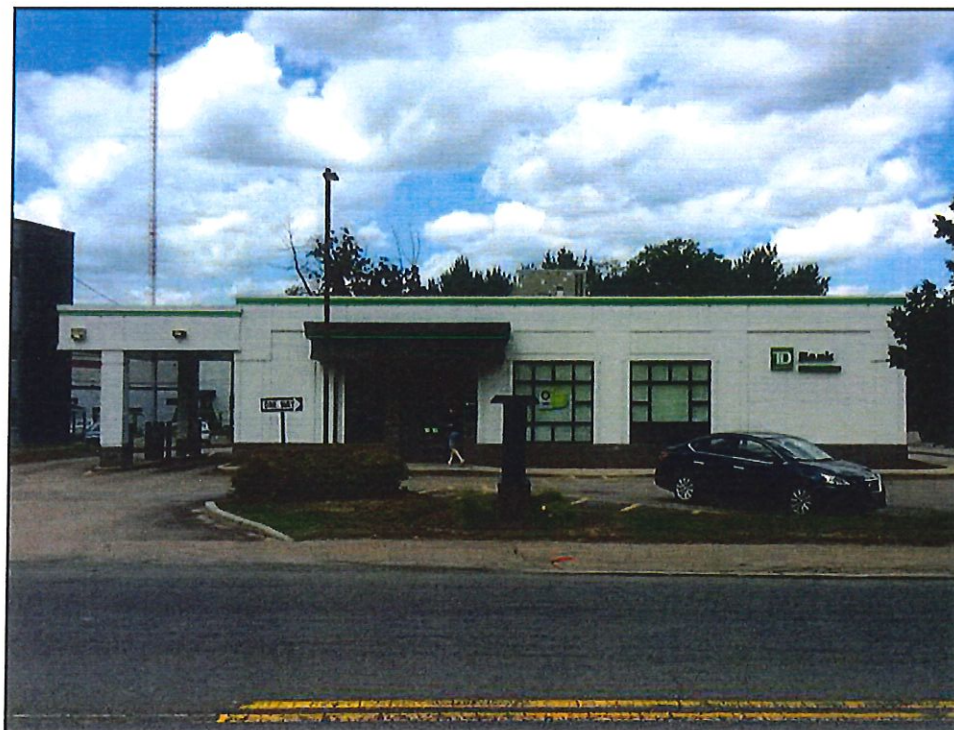
EXISTING SITE PHOTOGRAPH
