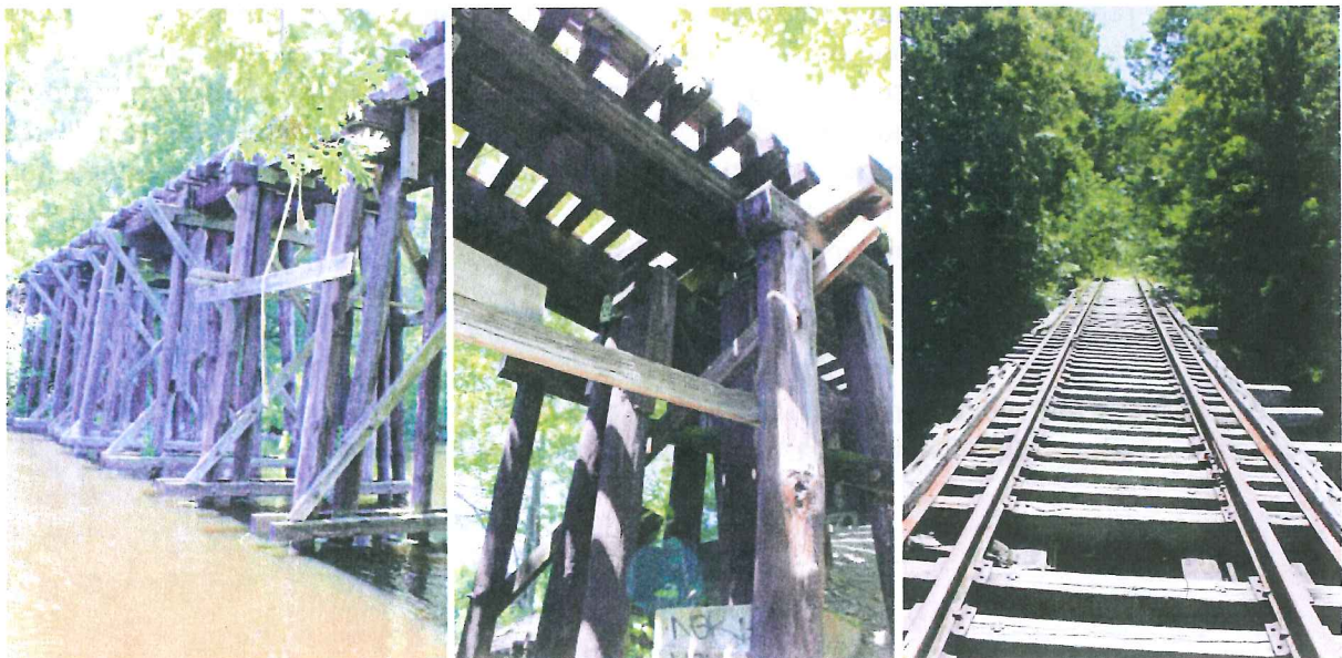
Views of the timber pile bridge crossing the Charles River
