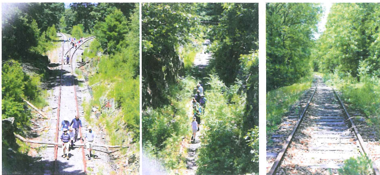
Views along the Needham section of the Bay Colony Rail Trail
