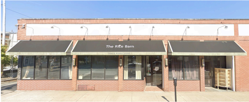
1 EXISTING EXTERIOR PHOTOGRAPH Scale: 1/4" = 1'-0"
