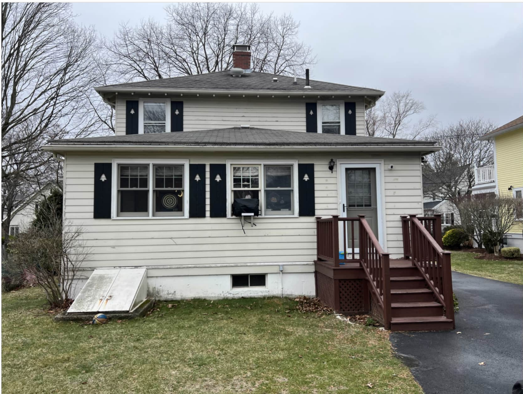
BACK FACADE (SOUTH ELEVATION)
