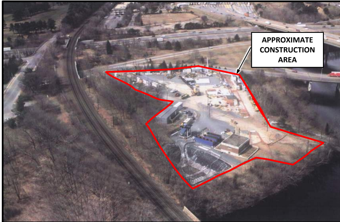
MWWST Shaft 5A – During Construction
