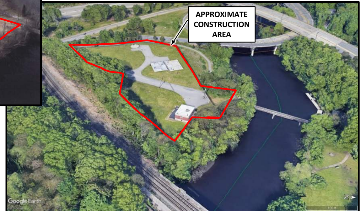
MWWST Shaft 5/5A – Post Construction
