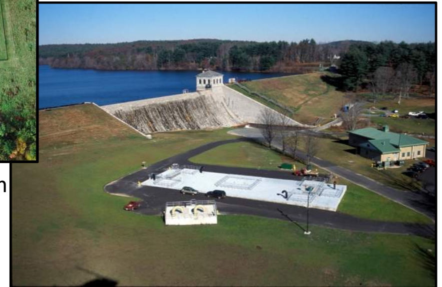
MWWST Shaft E, Southborough
