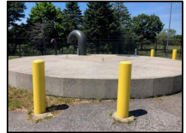
MWWST Shaft 5/5A, Weston
