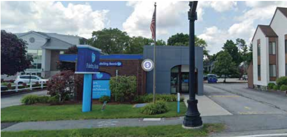
Building to right
