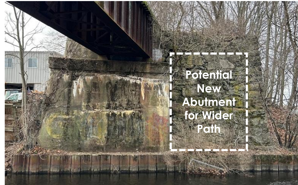
Existing West Substructure
