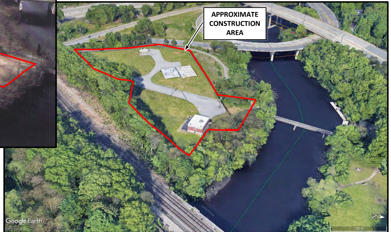
Shaft 5/5A – Post Construction
