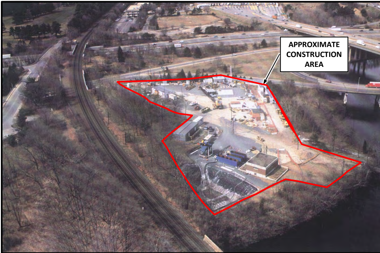
MWWST Shaft 5A – During Construction
