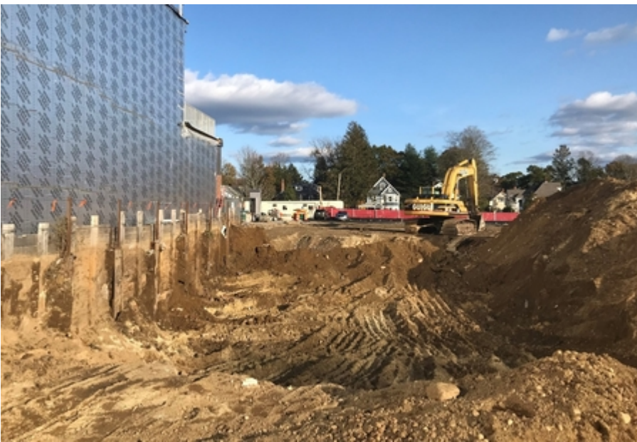
Excavation at Phase line – Chestnut Street
