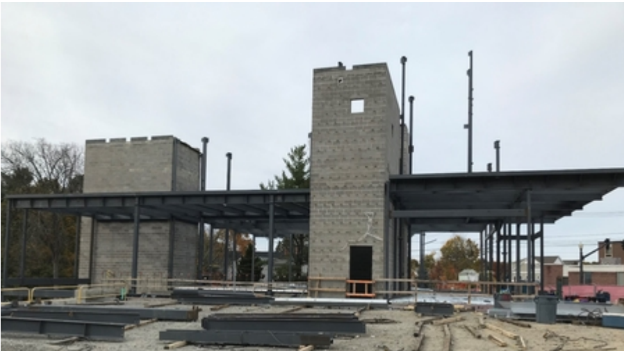
FS#2 Steel Erection second level
