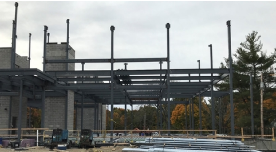
FS#2 Steel Erection
