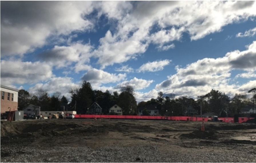
Chestnut St site after demolition of Public Safety
