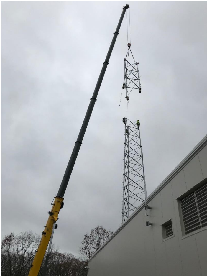
Communication Tower erection at Jack Cogswell Bldg/RTS
