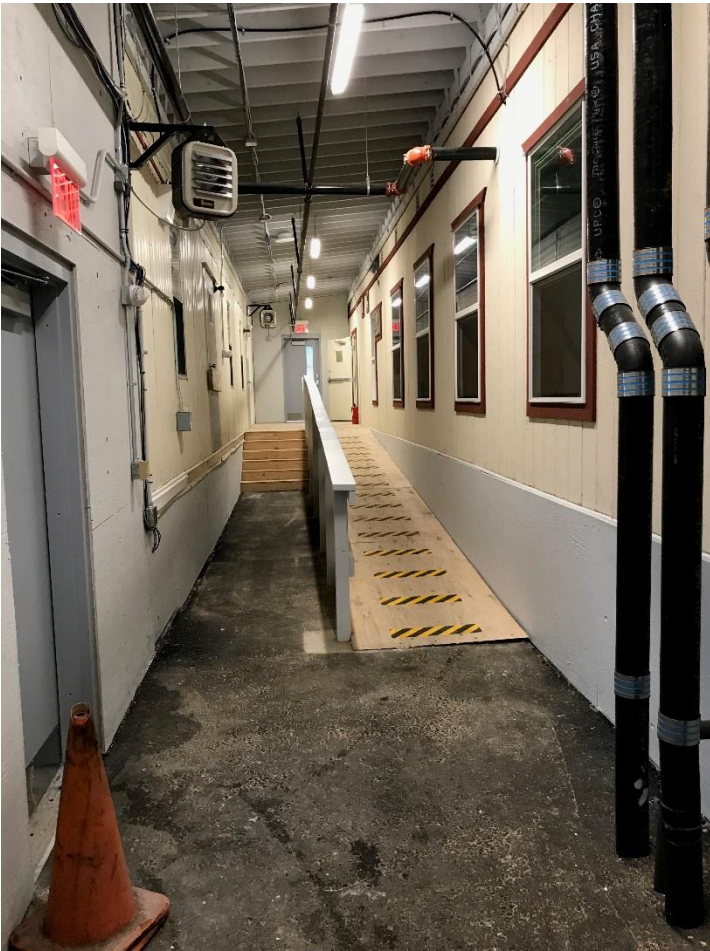
Temporary Fire Station #2 – Living Quarters
