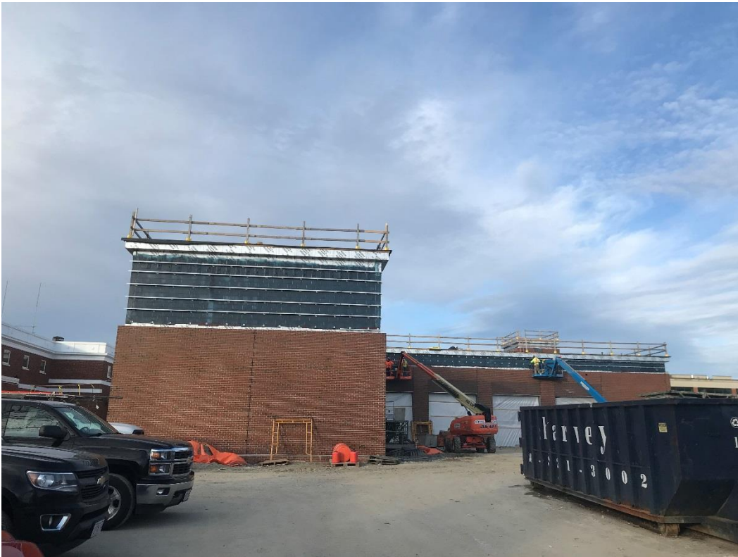
Fire Station #1 - East Elevation
