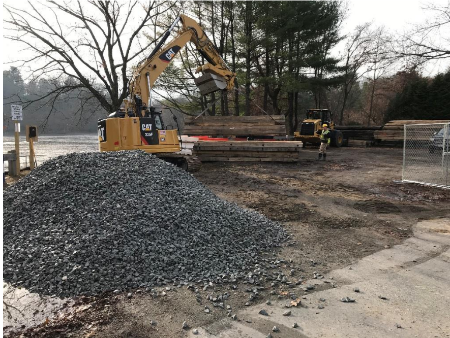
Gravel for Staging Area
