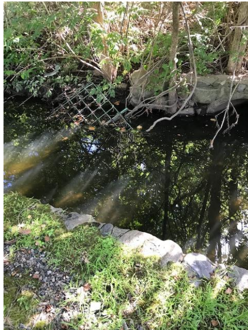
Station 2 (West Street) – Station similar to previous monitoring events. (9/5/2019)
