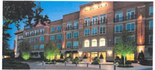
Charles River Landing Needham Permitting 350 rental units
