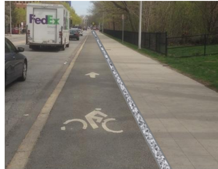
EXAMPLE of raised bike lane
