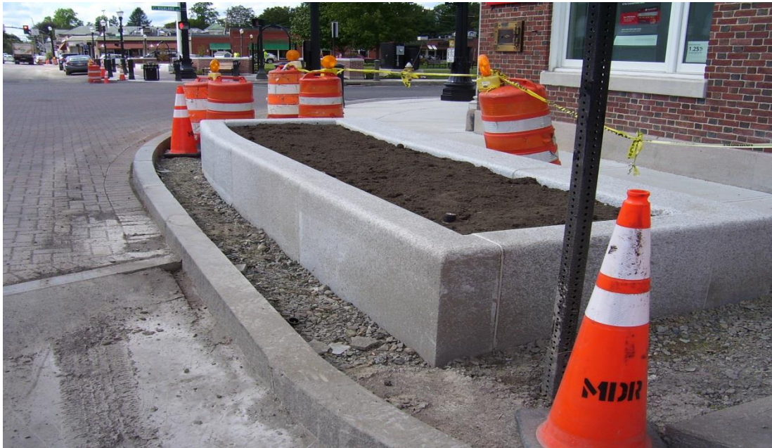
Final granite planter installed on the northeast corner of Great Plain Ave. and Highland Ave.
