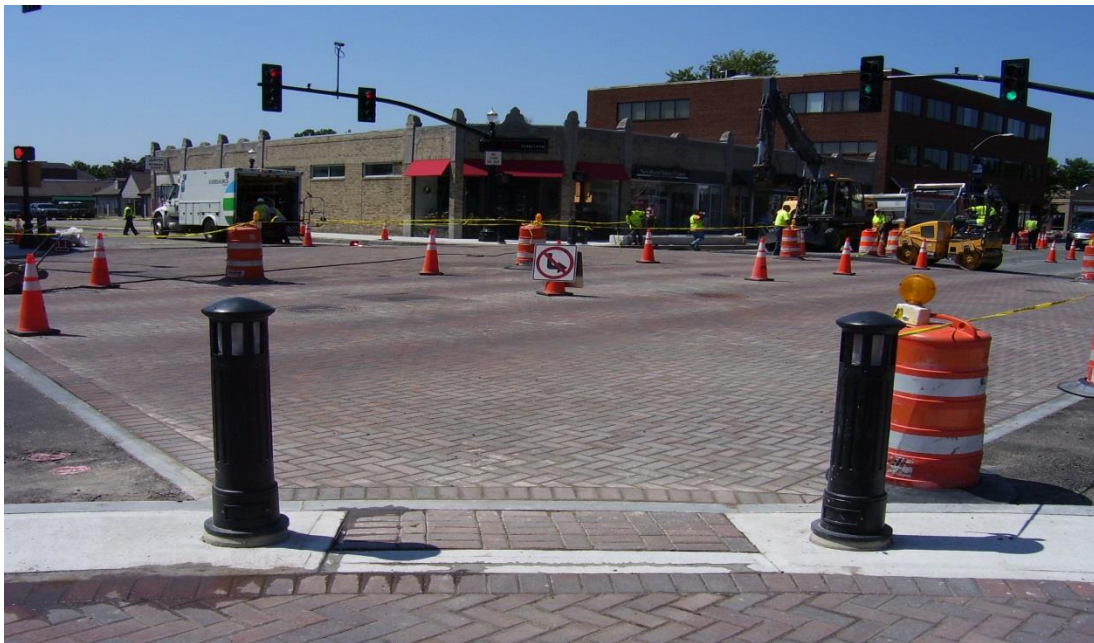
Completed brick paver crosswalk in Great Plain Ave. at the intersection of Chestnut St. and Chapel St.
