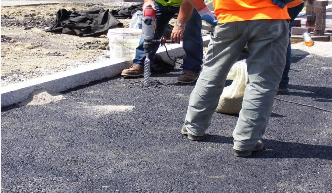
Drilling to construct weep holes in the asphalt base of the brick paver crosswalk
