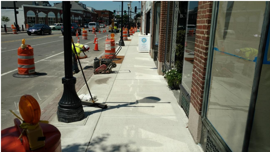
Paver Band Installation GPA
