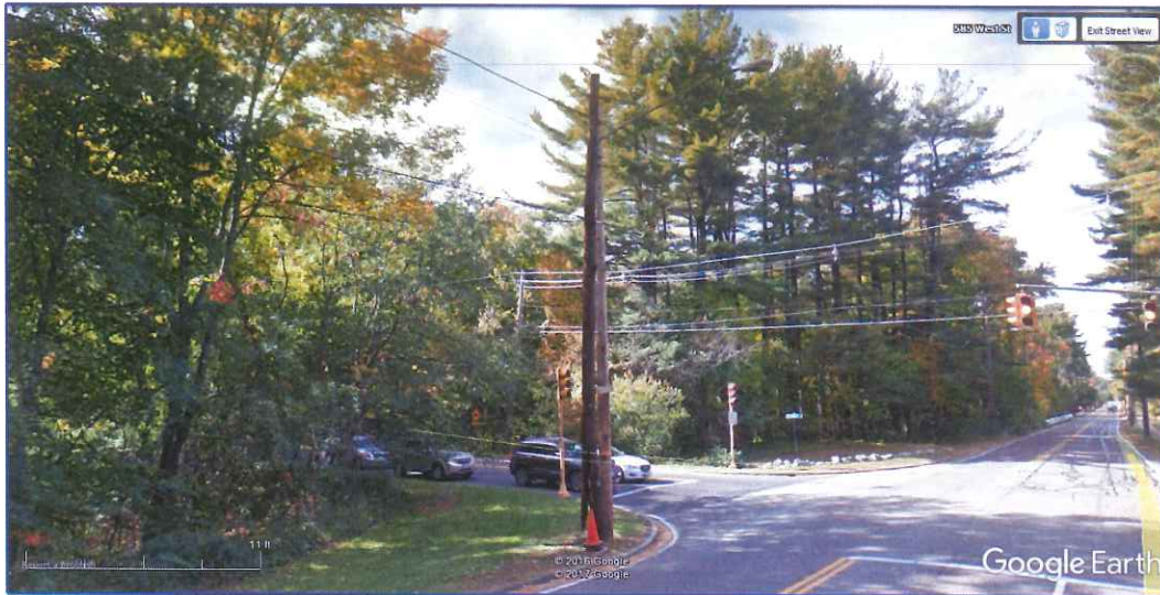
Figure 3G: Proposed Verizon Wireless Small Cell Antenna Site "Needham_MA_SC09"
