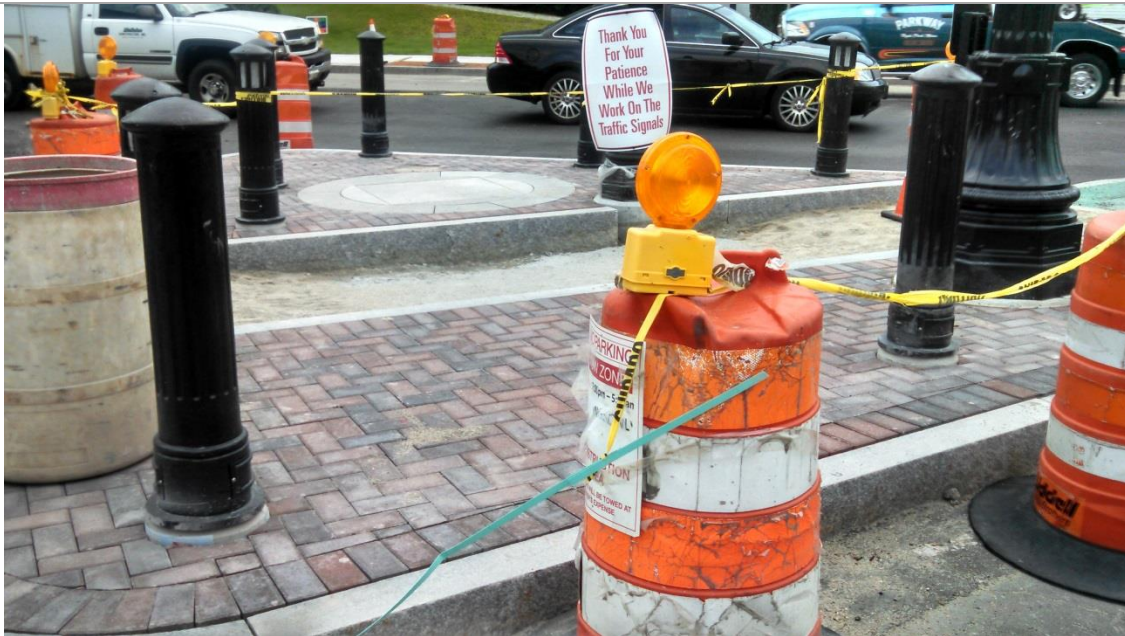
Dedham Ave. island with granite and brick pavers installed
