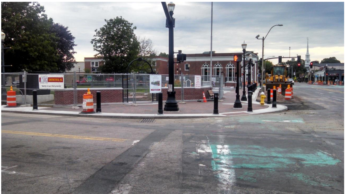
Front of Common looking west to east about 90% complete
