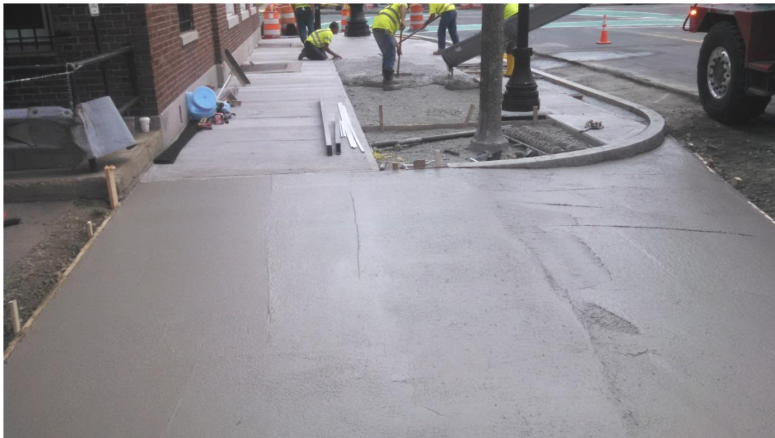
Placing concrete sidewalk in Highland Ave. in front of Santander Bank
