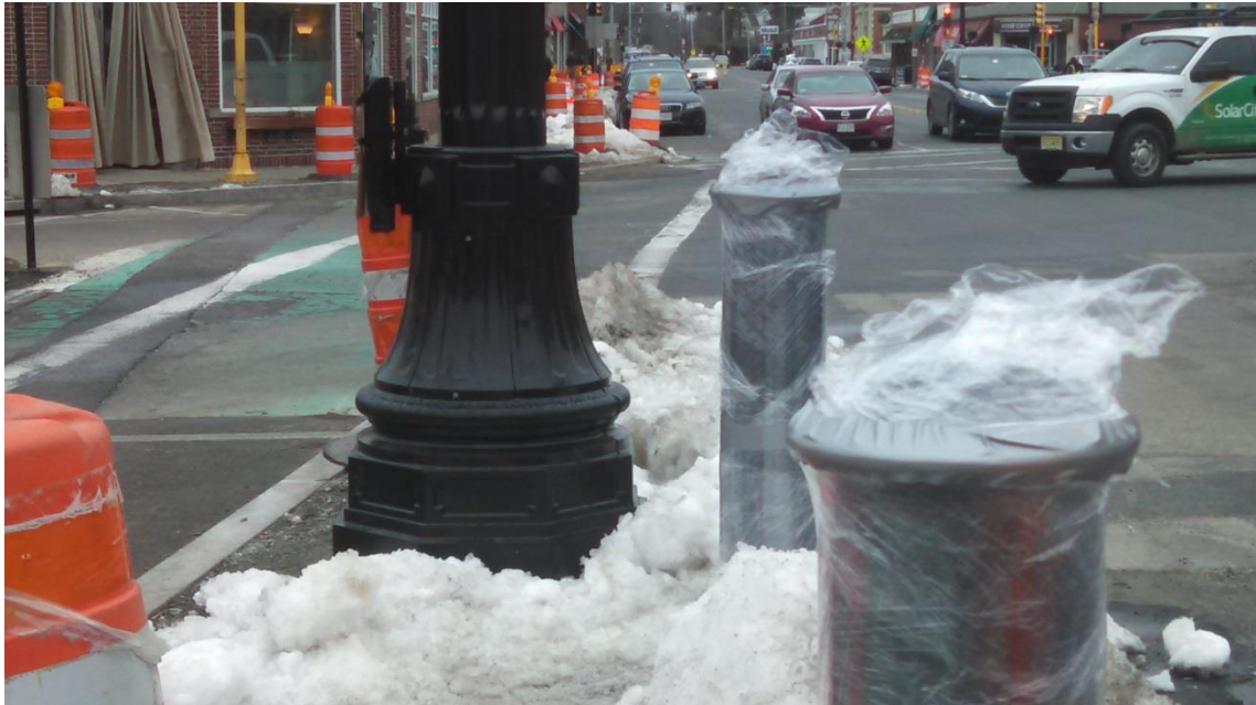
Pedestrian signal pushbutton and bollards installed in the Dedham Ave. island
