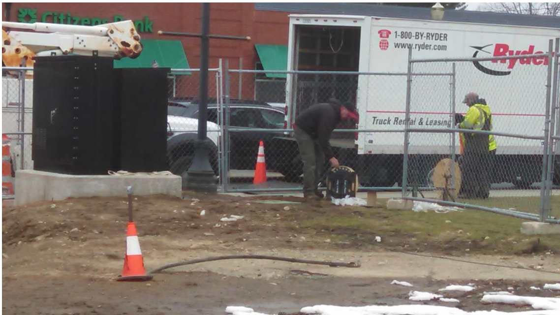
Installing wiring to the traffic and electrical controllers near Chapel St.
