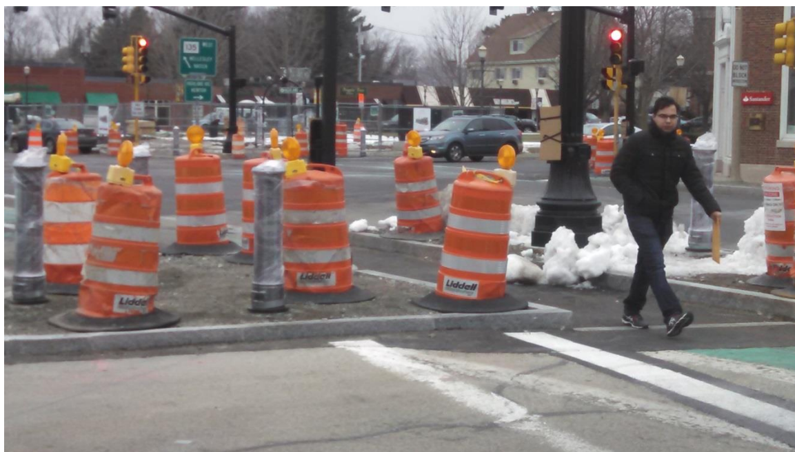
Bollards installed in the Dedham Ave. Island
