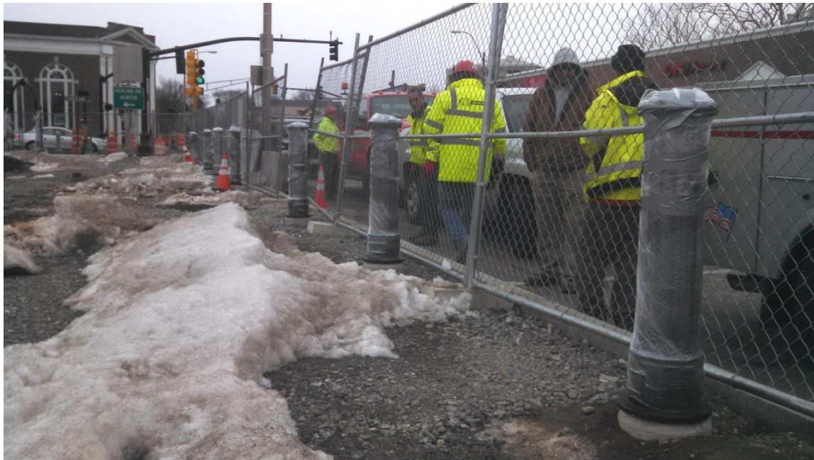
Bollards installed in front of the common
