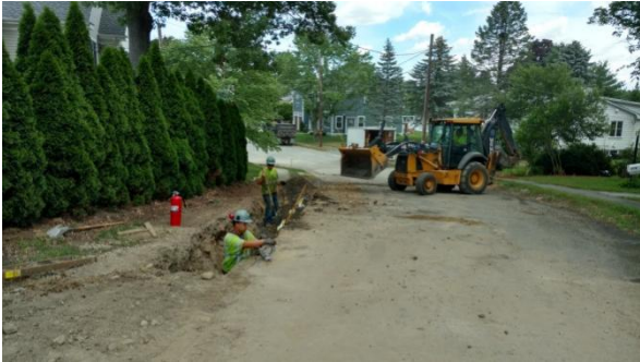
Feeney Bros. installing gas main Rockwood Lane (adjacent to #85 Richard Road)
