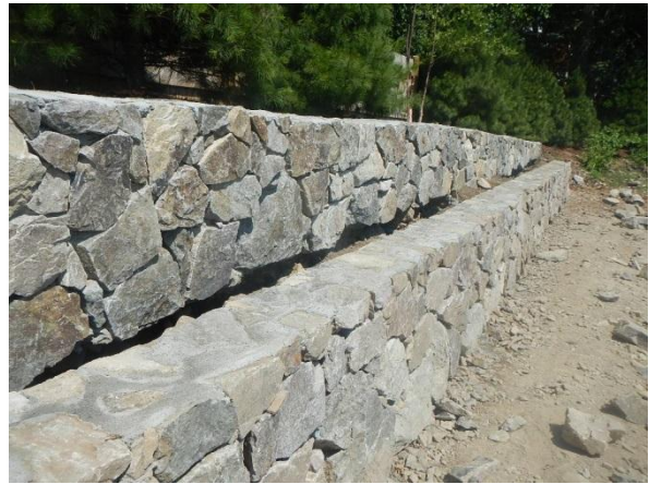
Planter wall along rear of Lot 5
