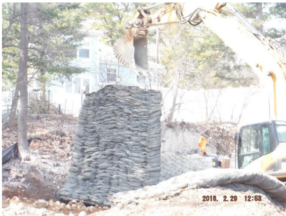
Blasting mats being set in place prior to first blast 2/29/16
