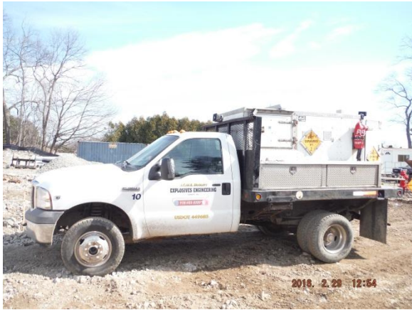
BCME Blasting on site blasting ledge Lots 2 & 3 2/29/16 - 3/2/16
