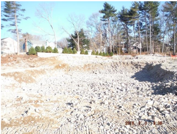
Foundation hole excavated for house Lot 4
