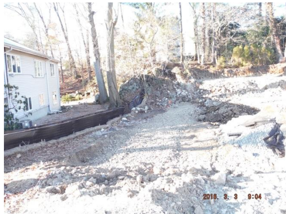
Foundation base prepped for retaining wall Lot 2 3/2/16
