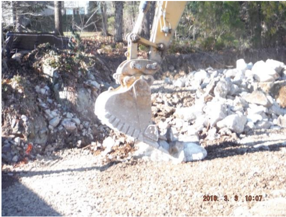
Titan Contractors providing blasted rock for wall building 3/3/16
