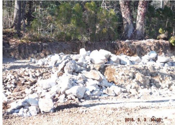
Stockpile of blasted rock Lot 1 for retaining wall 3/3/16
