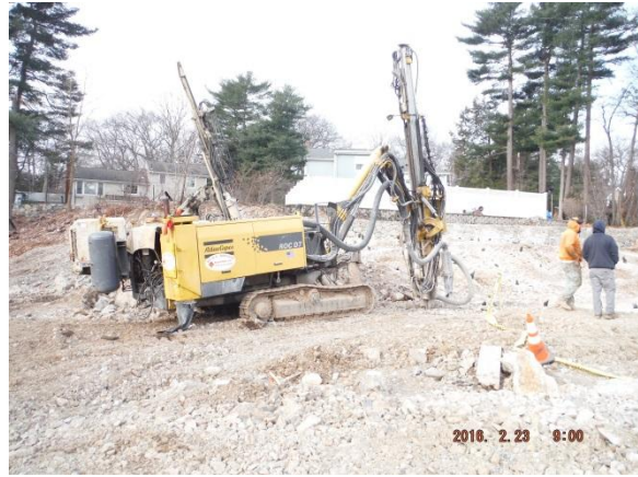
Drilling continues Lots 2 & 3 as needed 2/29/16 - 3/2/16
