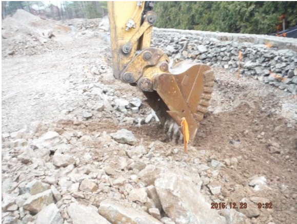
Titan removes fill from area around CB 3 12/23/15
