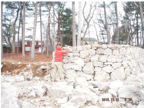
WSW Masonry completes stone wall northwest section of Lot 6 - 12/21/15
