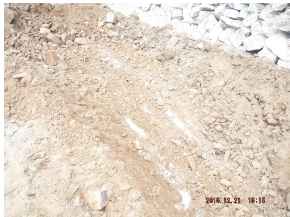
Ledge encountered installing underdrain Lot 7 - 12/21/15
