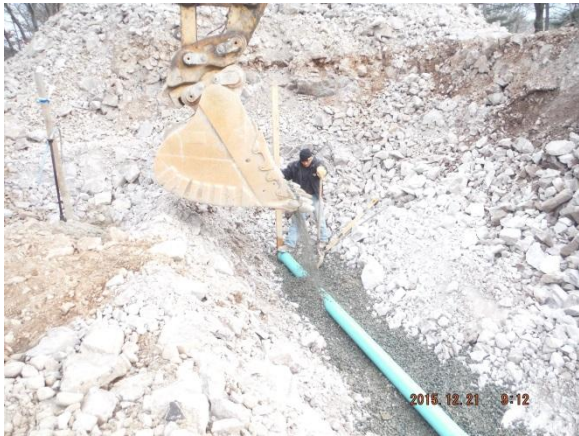
Titan extends sewer service Lot 6 - 12/21/15
