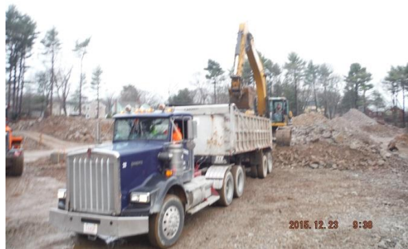
Independent truckers hauling blasted rock of site 12/21/15 – 12/23/15
