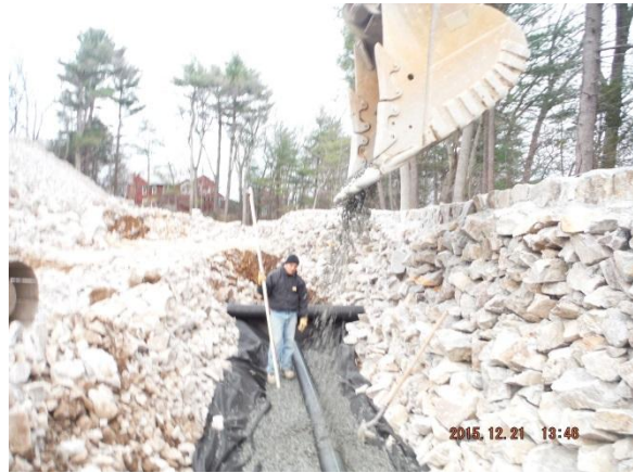
Titan extends underdrain Lot 8 & Lot 7 - 12/21/15
