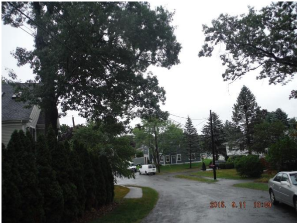
Overhead wires repaired at 30 Rockwood Lane
