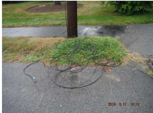
Wires cut from poles and left at curb
