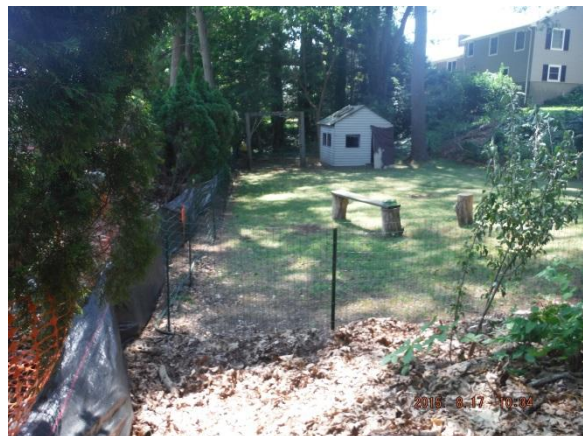
Silt fence installed behind stockpile and fence repaired behind 63 Tudor Road.
