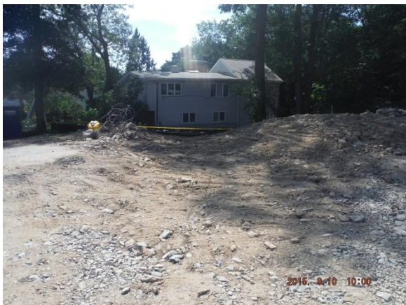
Stormwater runoff swale installed 8/10/15
