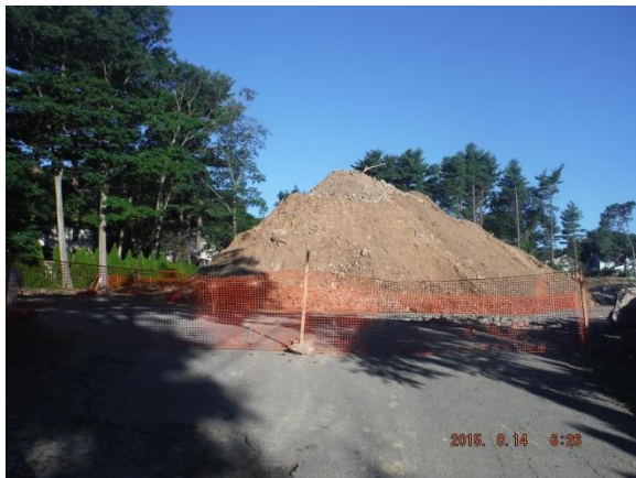
4' temporary plastic fence installed around perimeter of stockpiled material
