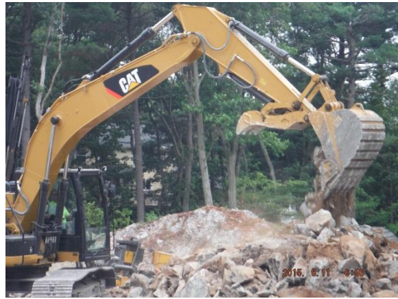
Blasted rock excavation continues
