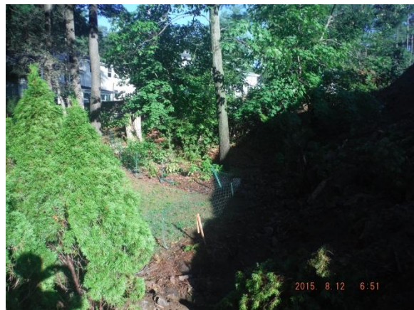
Boulders removed from rear of property located at 63 Tudor Rd
