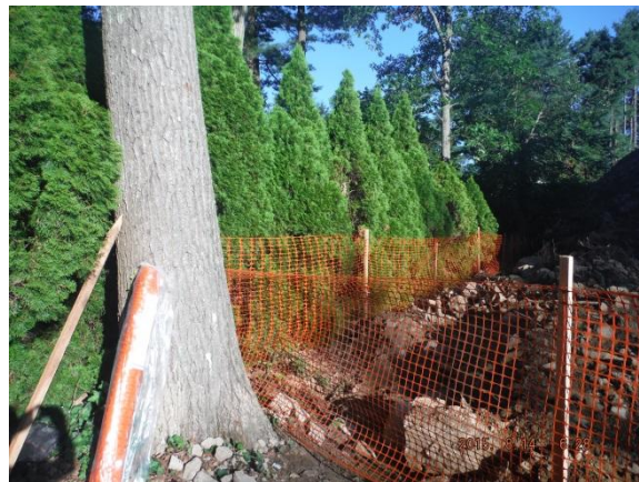
Temporary fence installed around back of stockpile behind 63 Tudor Rd.
