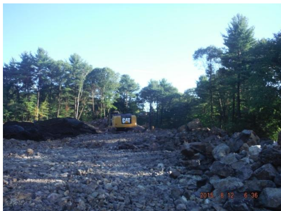
View of site surface after blasting
