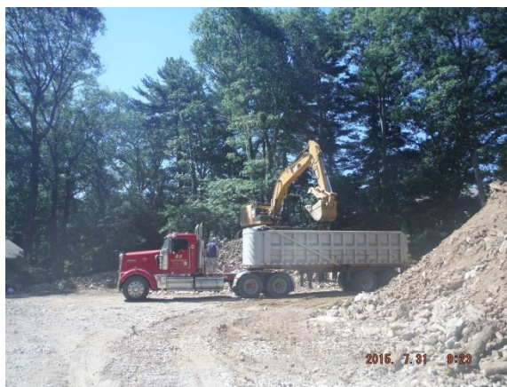
Trailers hauling excavated rock and soil offsite to Tresca Brothers Concrete
