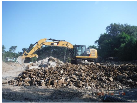
Excavation of blasted rock
