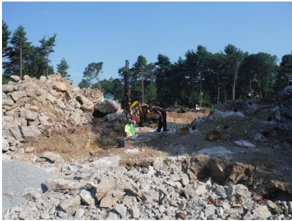
Rock Drilling Continues Daily
