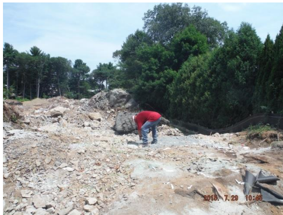
Loading holes for first blast 7/29/15
