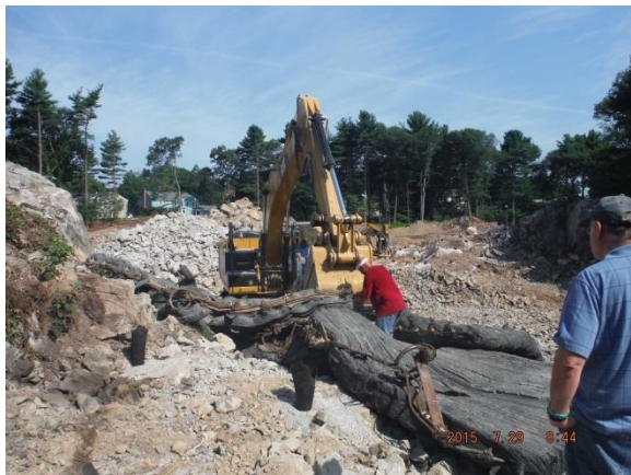
Setting blasting mats prior to blasting
