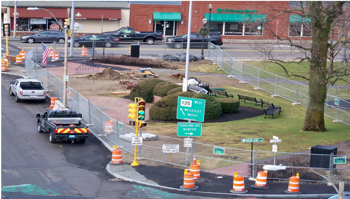
Photo of Common area where new landscape/hardscape features will be constructed
