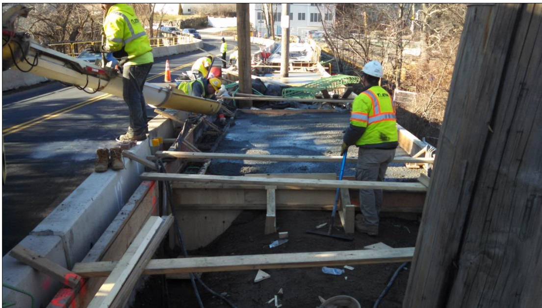
Pouring Concrete for Northeast Approach Sidewalk 12/21/2016
