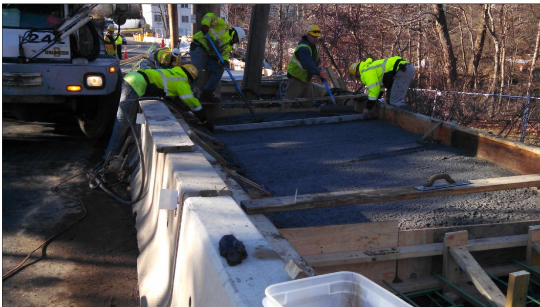
Pouring Concrete for Northeast Approach Sidewalk 12/21/2016
