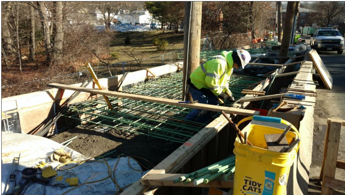
Installing Reinforcement for Northeast Approach Sidewalk 12/20/2016
