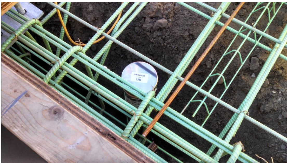
Time Capsule Placed within Northeast Approach Sidewalk Concrete Pour 12/21/2016
