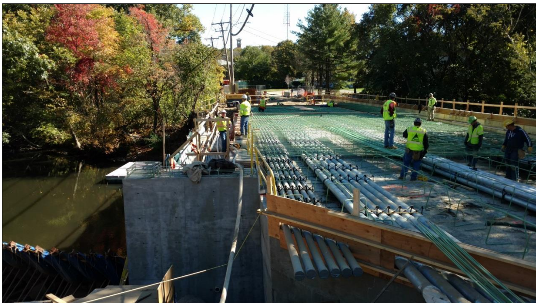
Installing Reinforcing Steel for Top Lift of Arch Saddle 10/11/2016
