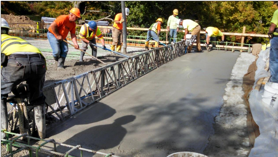
Pouring and Screeding Concrete for Top Lift of Arch Saddle 10/13/2016
