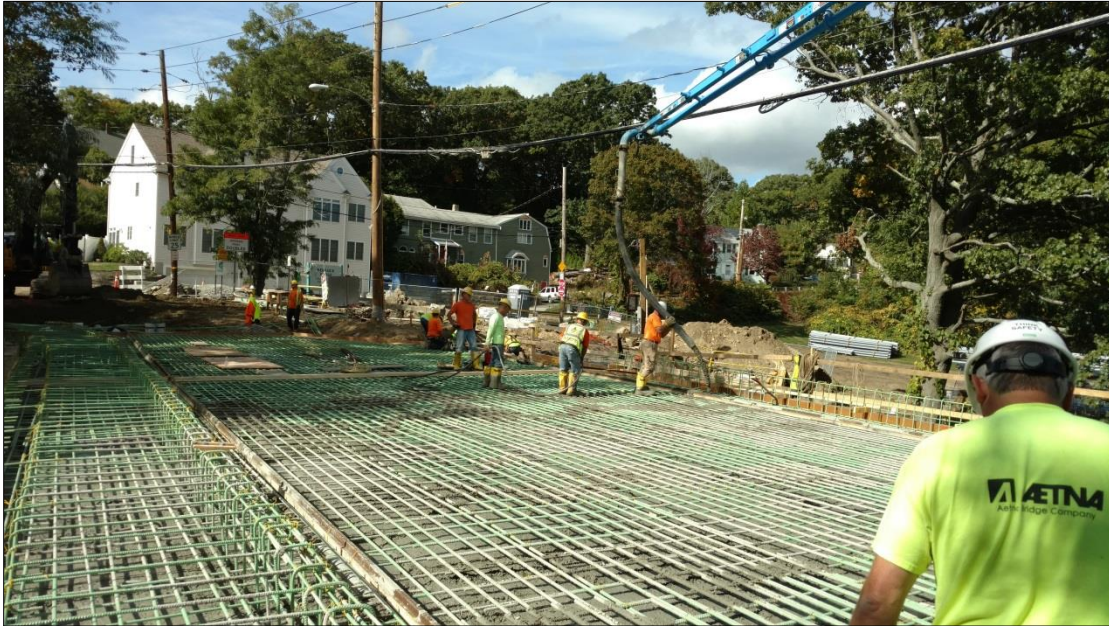
Pouring Concrete for Top Lift of Arch Saddle 10/13/2016
