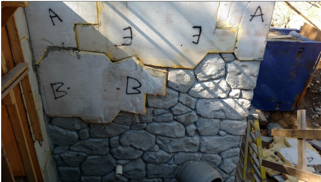
Partially Stripped Form Liner at Northwest Wingwall 10/11/2016
