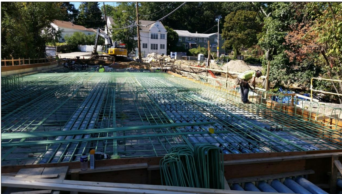
Installing Reinforcing for Top Lift of Arch Saddle 10/7/2016
