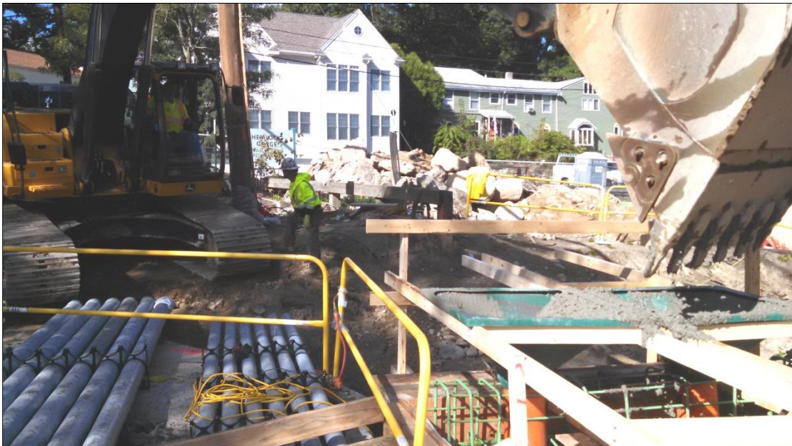
Transporting Concrete to Northwest Wingwall via Excavator Bucket 10/05/2016
