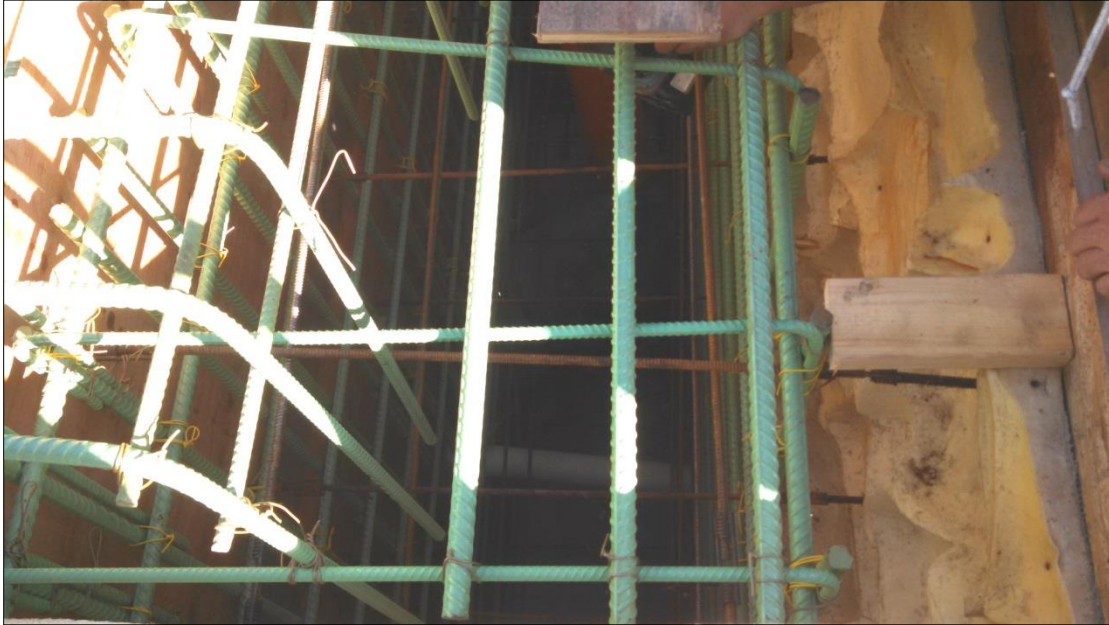
Looking Down into Formwork for Northwest Wingwall 10/05/2016
