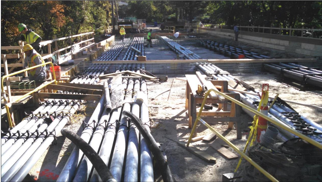
Installing Bulkheads and Reinforcing for Top Lift of Arch Saddle 10/5/2016
