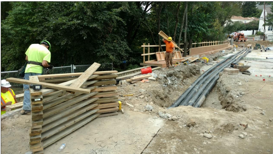
Installing Formwork for Southeast Spandrel Wall and Sidewalk 9/23/2016
