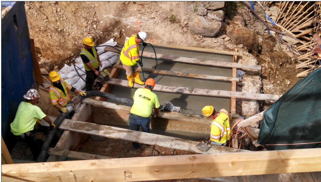
Pouring Concrete for Mud Slab at Northwest Wingwall 9/21/2016
