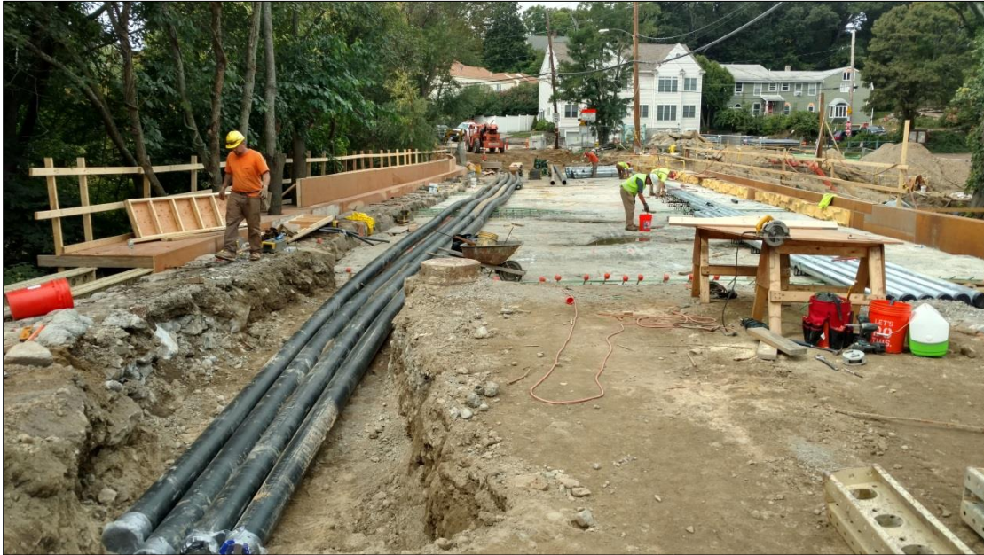
Installing Galvanized Steel Utility Conduit on Arch Saddle 9/23/2016
