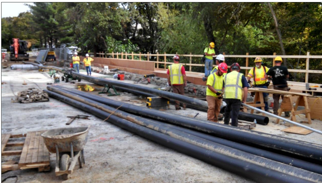
Installing HDPE Utility Conduit on Arch Saddle 9/21/2016
