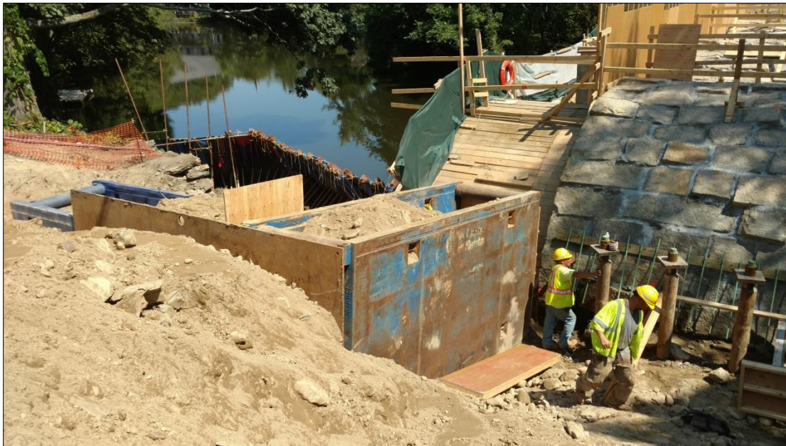
Temporary Excavation Support at Northwest Wingwall 8/24/2016
