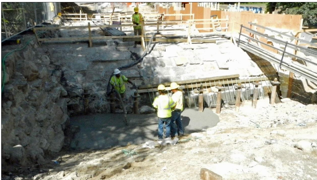
Pouring Base Concrete Saddle Pour at East Abutment 8/25/2016
