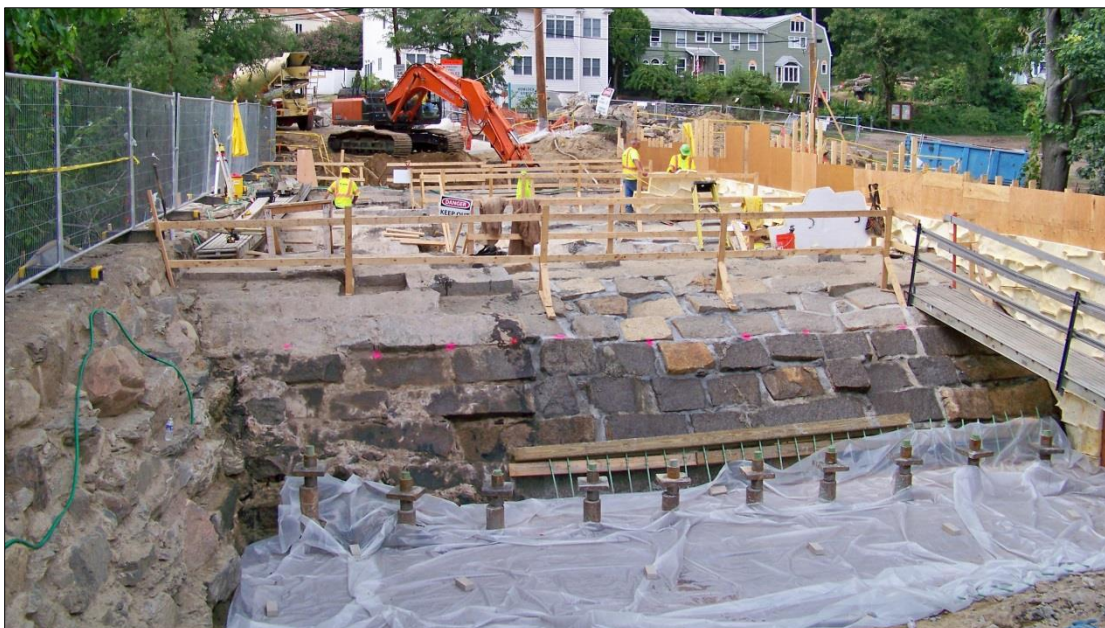
Curing Base Pour of Arch Saddle Concrete at East Abutment 8/26/2016
