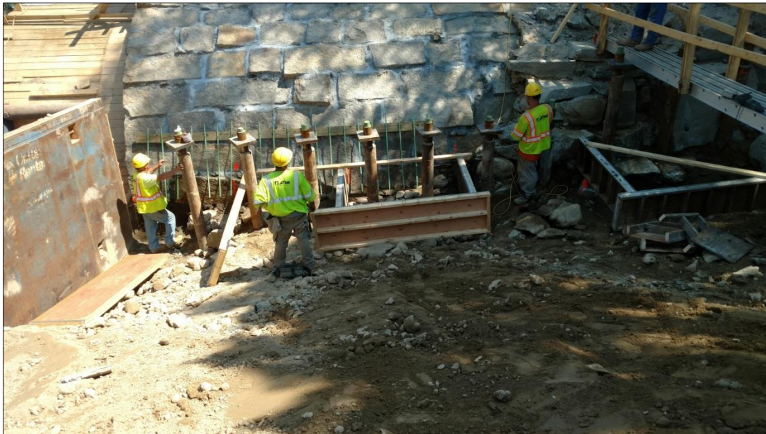
Installing Formwork and Dowels for Saddle Base Pour at West Abutment 8/24/2016
