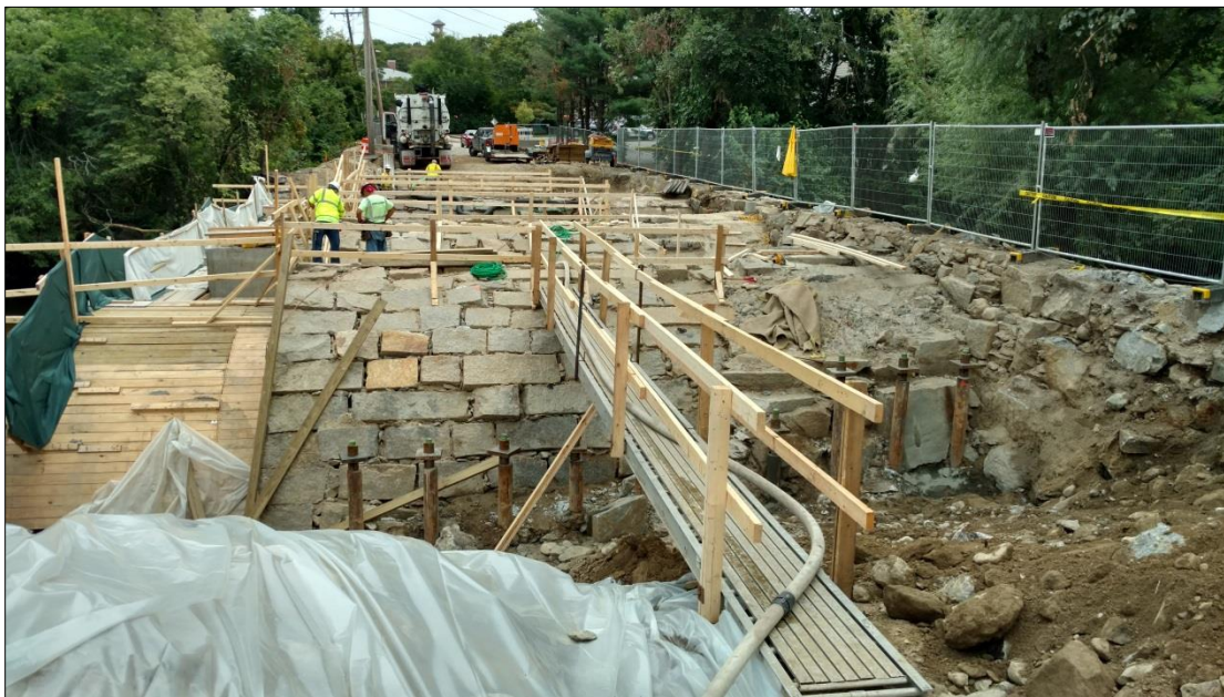
View of Arches Looking East 8/16/2016
