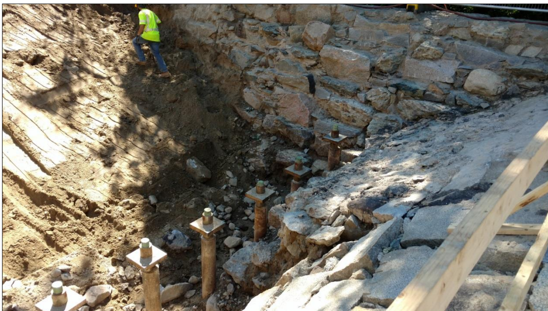
Cut Off Piles at East Abutment 8/18/2016
