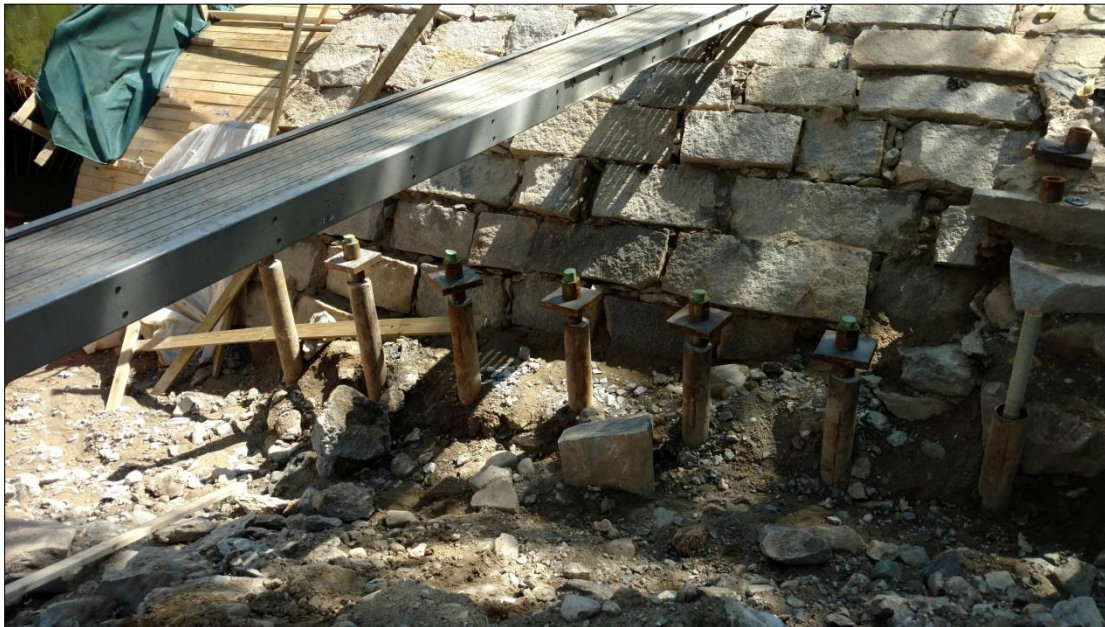
Cut-Off Piles at West Abutment 8/15/2016
