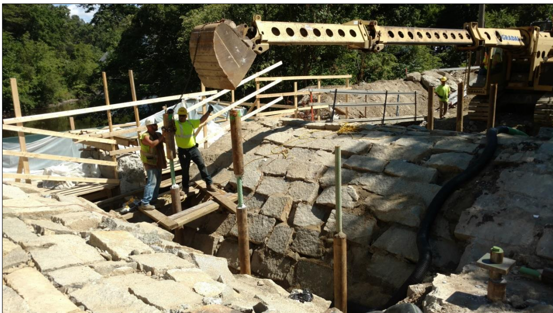
Cutting Off Piles at Pier 8/15/2016
