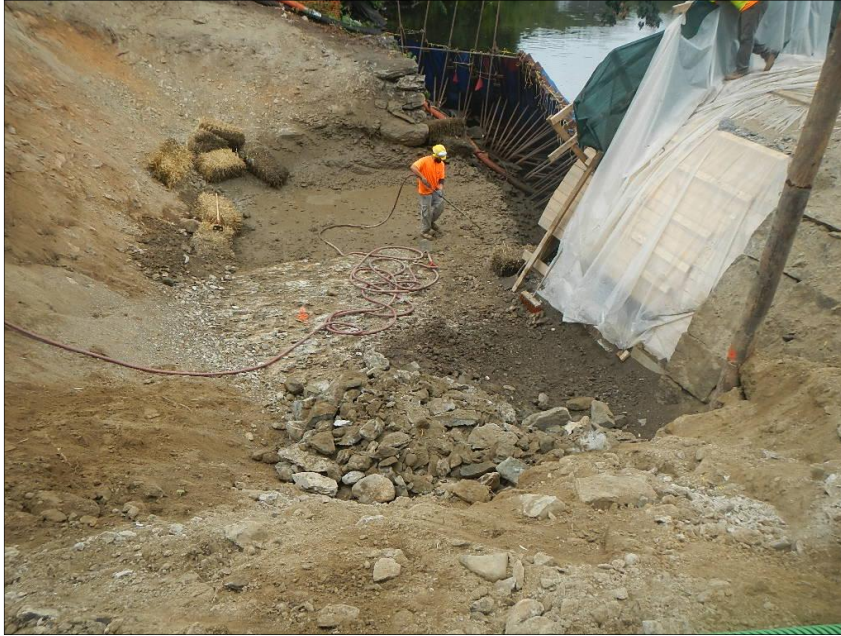
Top of Bedrock at West Abutment and NW Retaining Wall 8/10/16
