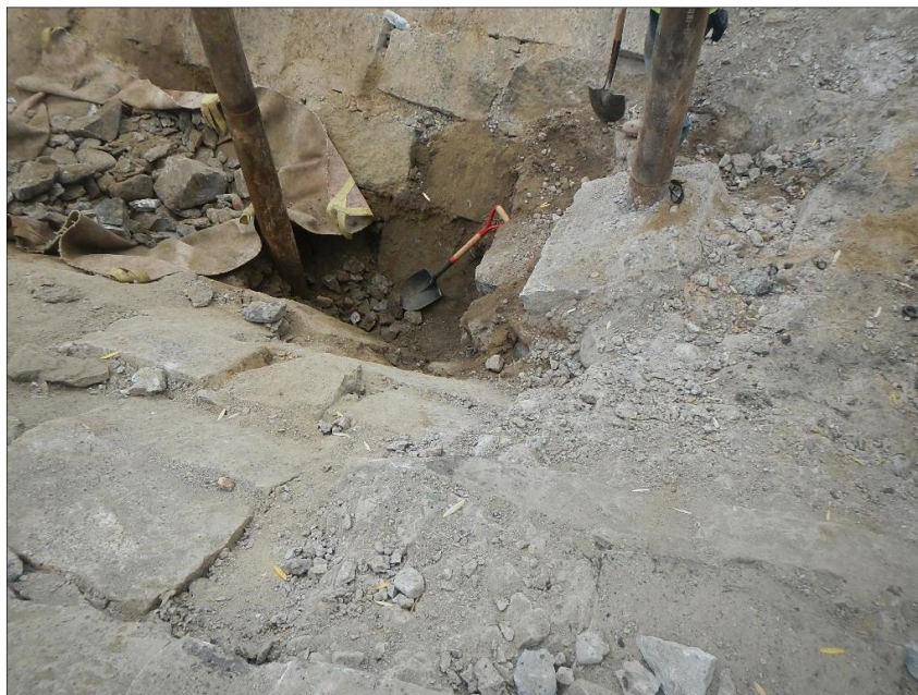
Partially Removed Concrete Fill at Pier Location 8/10/16
