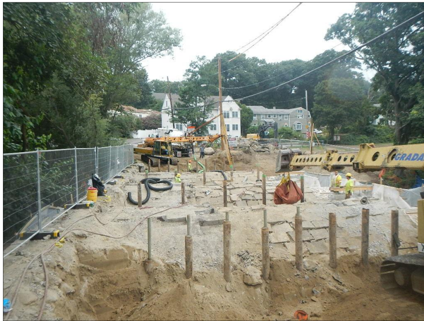
General Photo of Exposed Stone Arch 8/10/16
