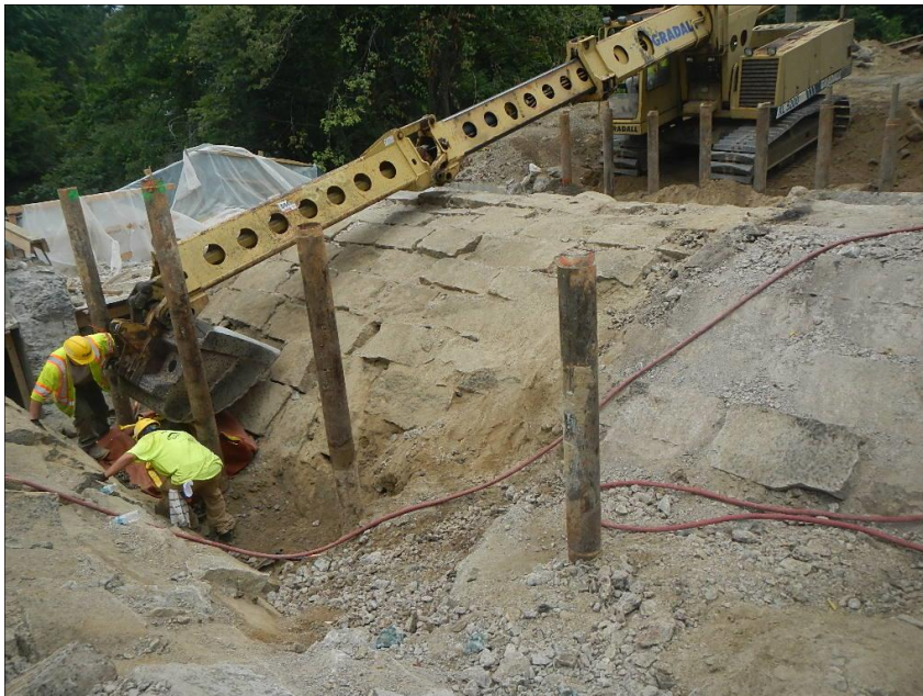
Arch Fill Removal at Pier 8/10/16
