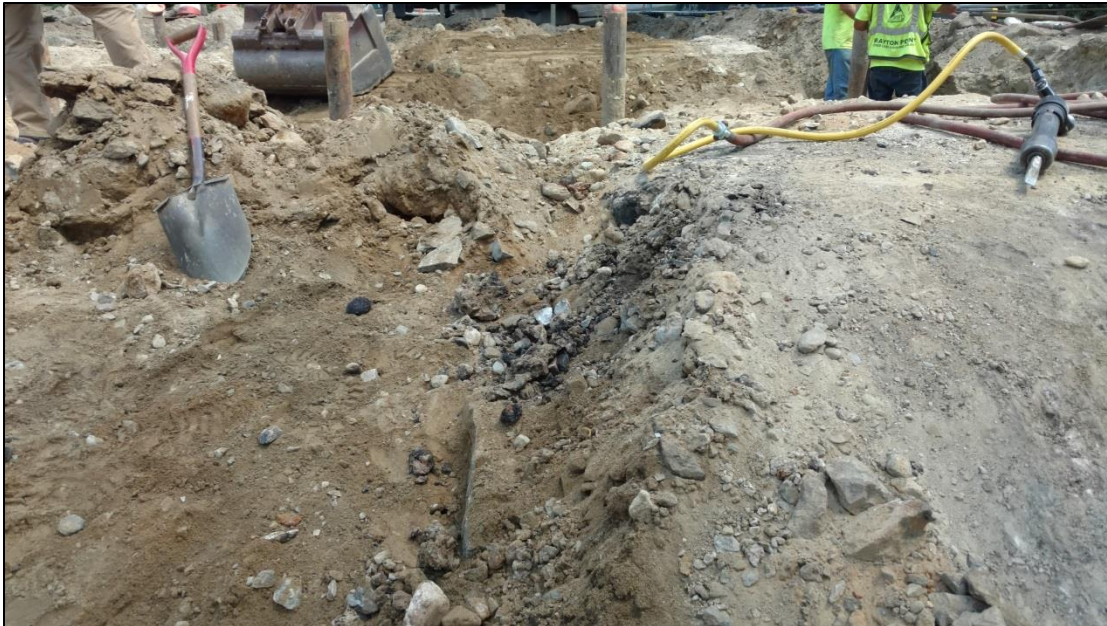
Excavation Adjacent to Concrete Course Covering Arches (Right) 8/4/2016
