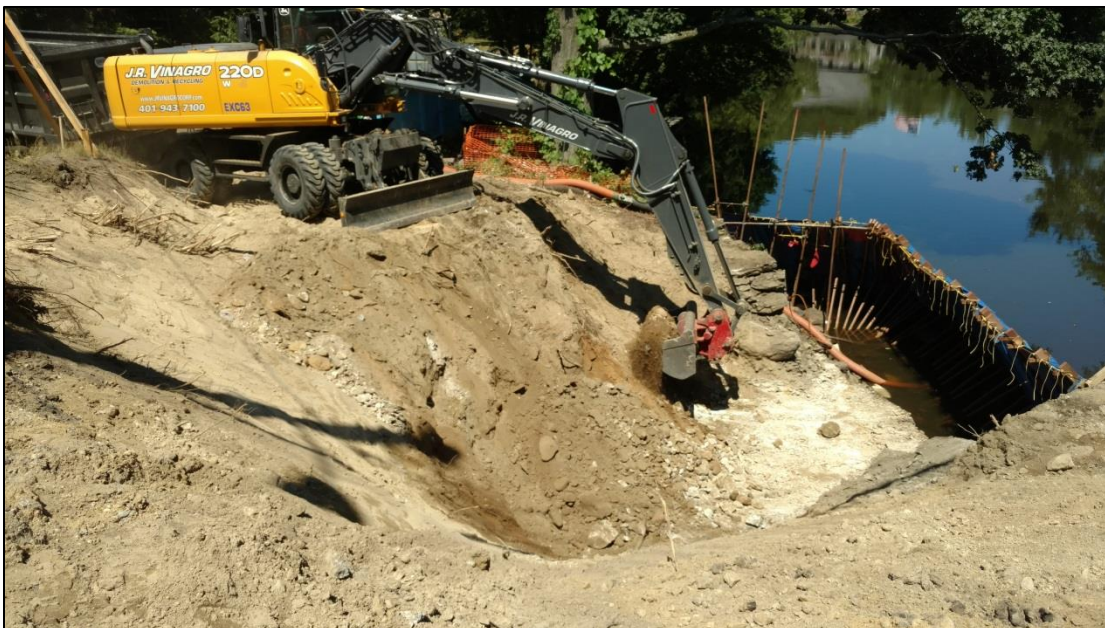
Excavation for Northwest Wingwall Footing 8/3/2016
