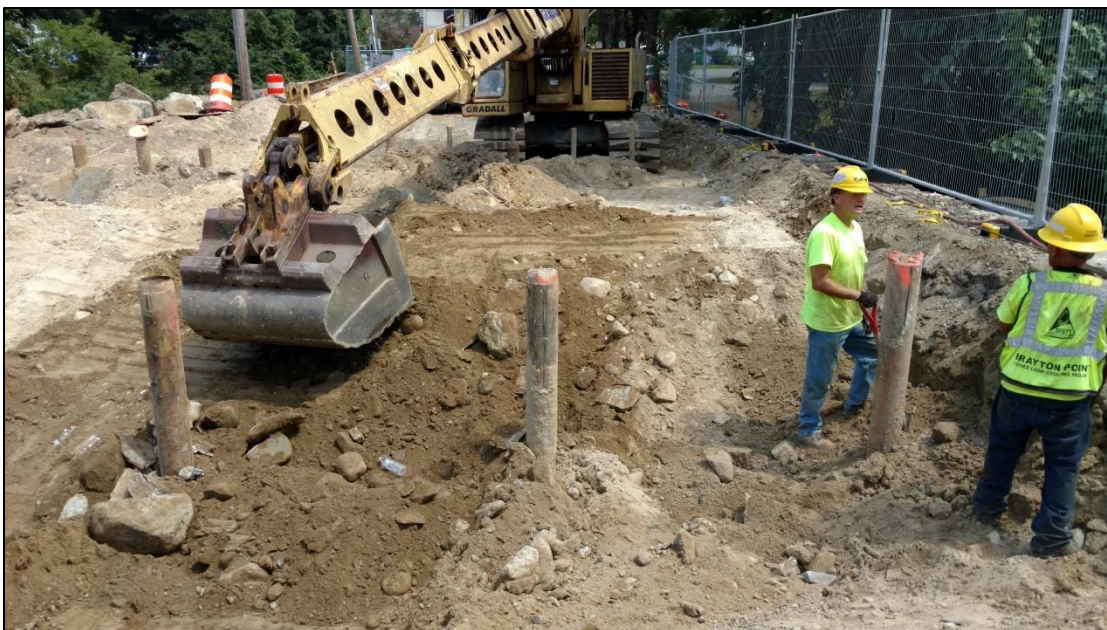
Excavation of Fill Between Arches and Micropiles 8/4/2016
