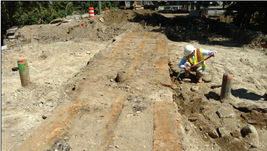
Steel Beams Uncovered During Excavation of Arch Fill 8/3/2016
