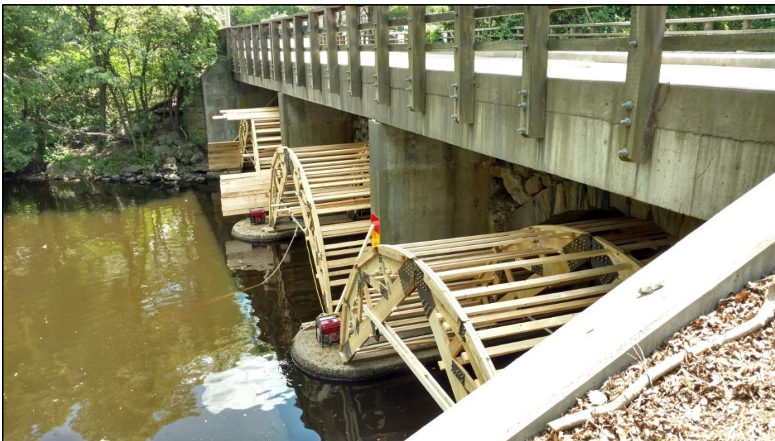
Progress of Temporary Arch Support Installation 6/20/2016
