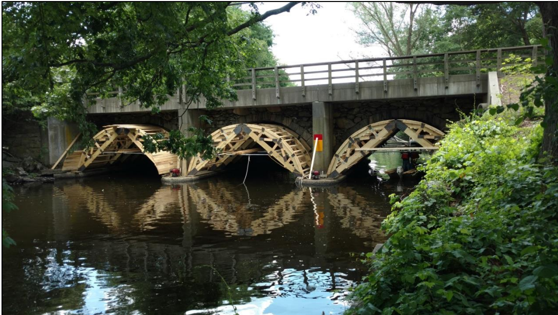
Progress of Temporary Arch Support Installation 6/20/2016
