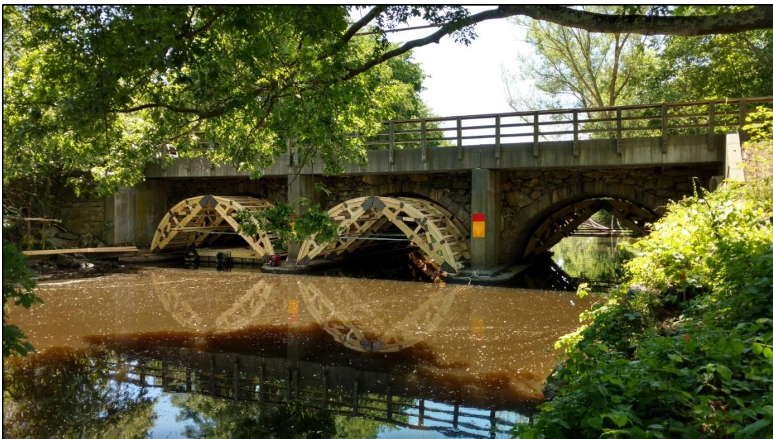
Progress of Temporary Arch Support Installation 6/17/2016
