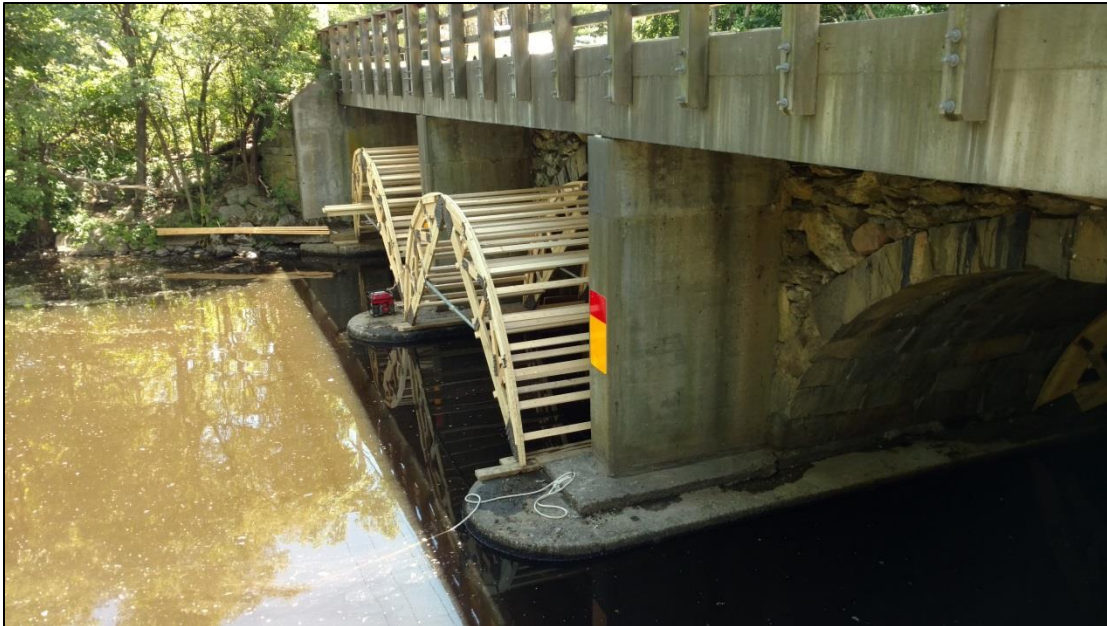
Progress of Temporary Arch Support Installation 6/17/2016
