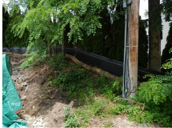
Previously Installed Silt Fence and Straw Wattles
