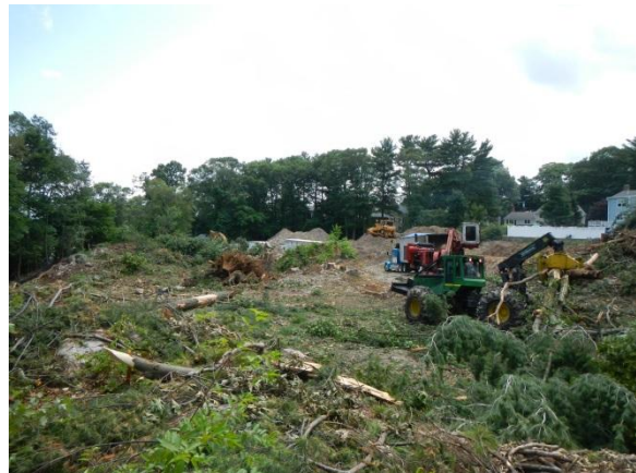
Site Clearing Underway
