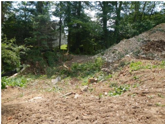
Removal of 4 Remaining Trees SW Corner of Site
